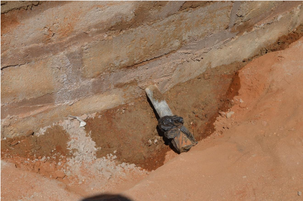
Figure 63: Tap positioning and installed on bottom course
