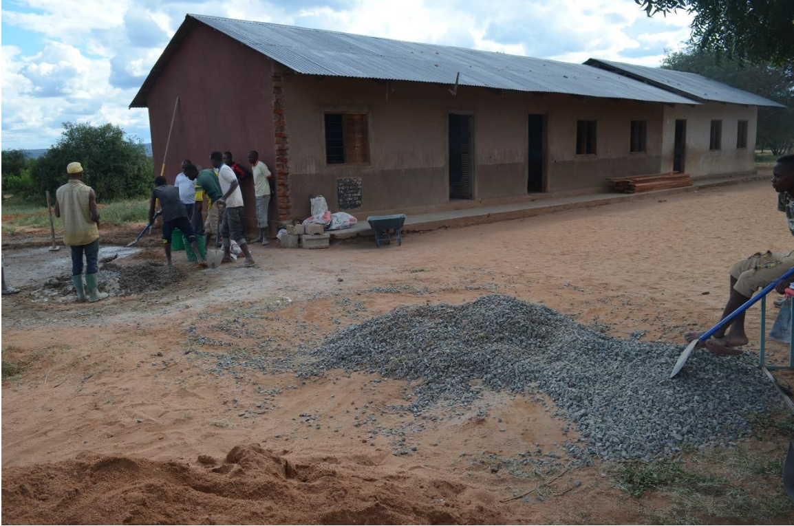
Figure 51: Remaining aggregate after foundation
