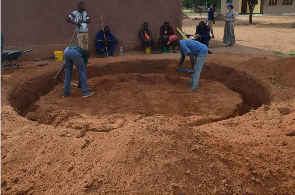
Figure 15: Completing Slab Excavation
