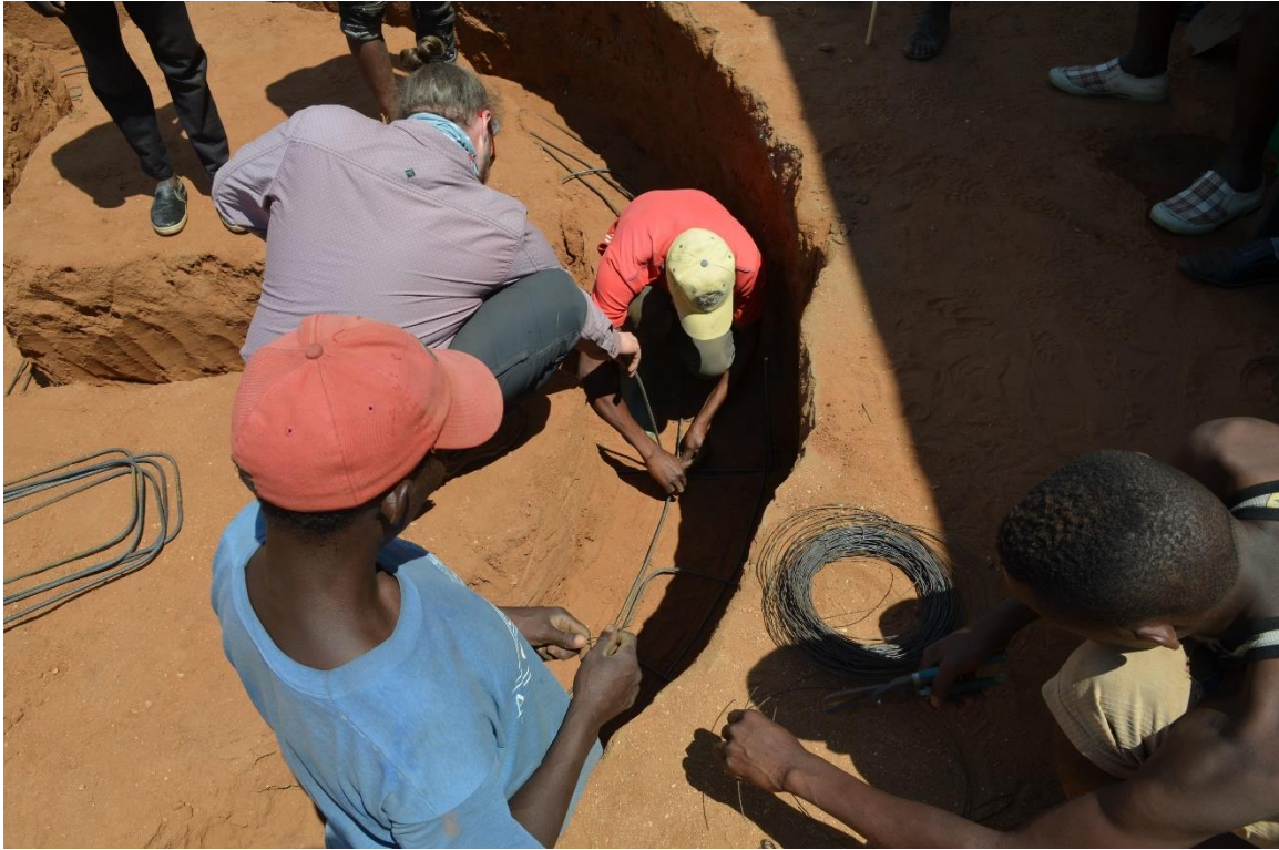
Figure 26: Tying of Stirrups and Footing Steel
