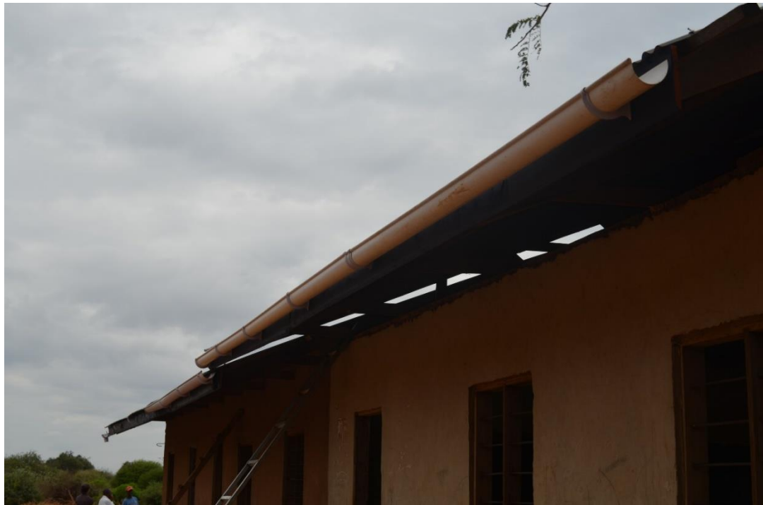
Figure 57: Gutter: higher side installed
