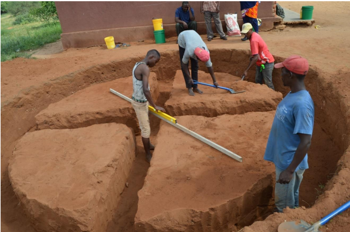
Figure 18: Finishing Beams and leveling
