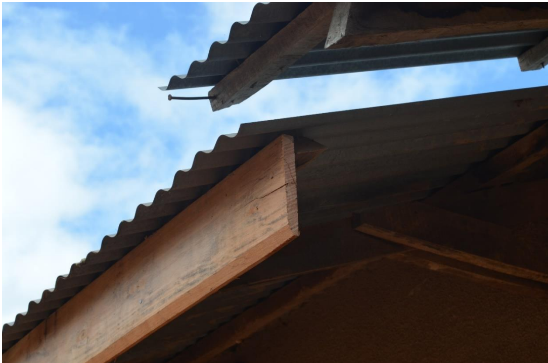
Figure 53: Close up of installed facia board
