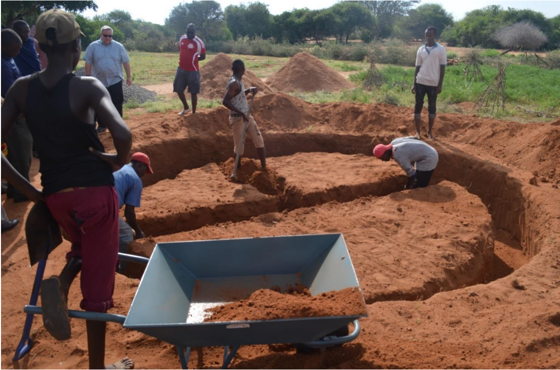
Figure 17: Foundation Beam Excavation
