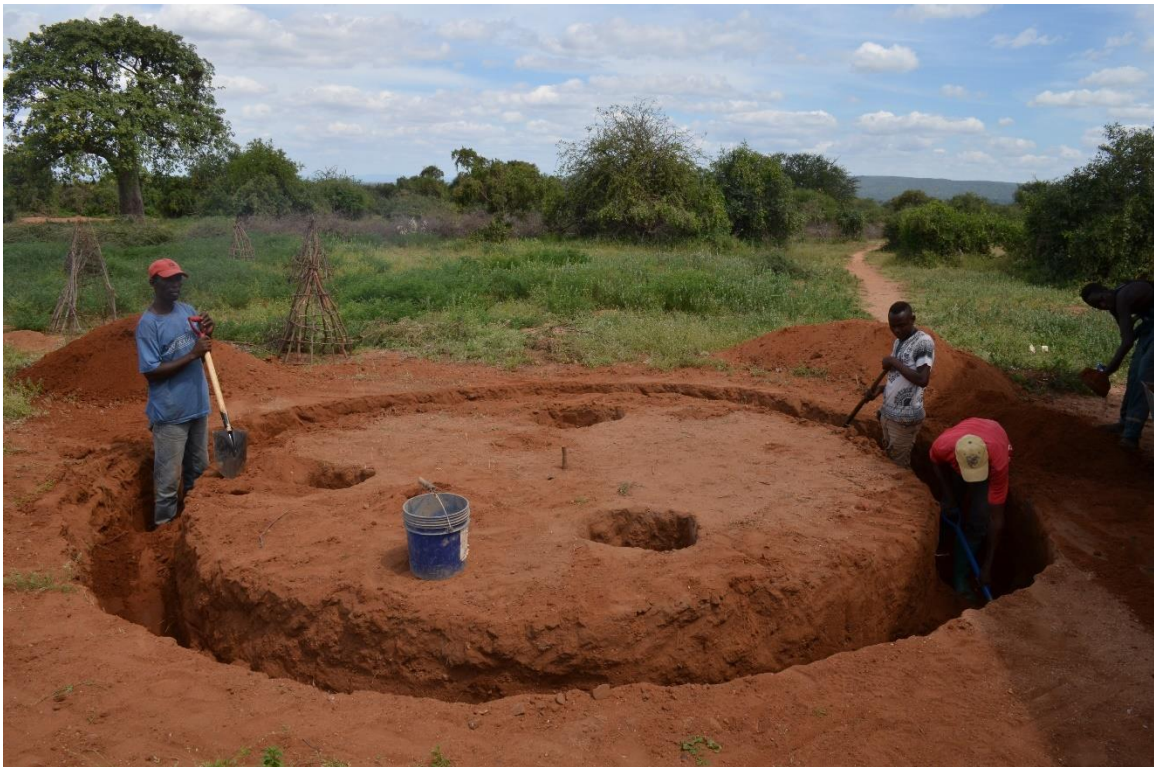
Figure 12: Finishing of the Footing
