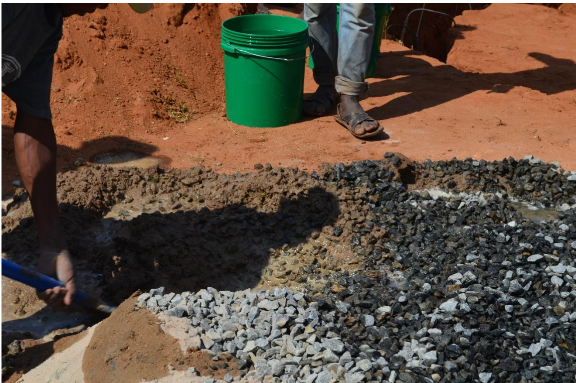
Figure 36: First Batch Mixing
