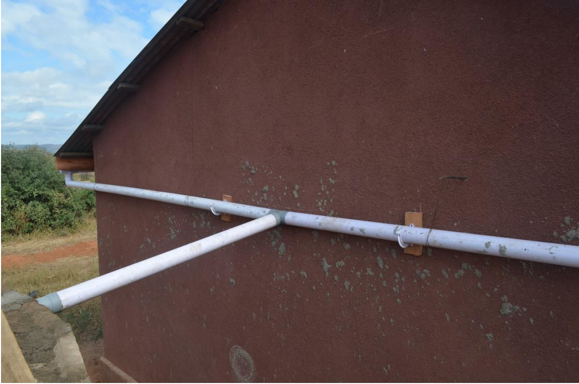
Figure 72: Piping to Tank Connections
