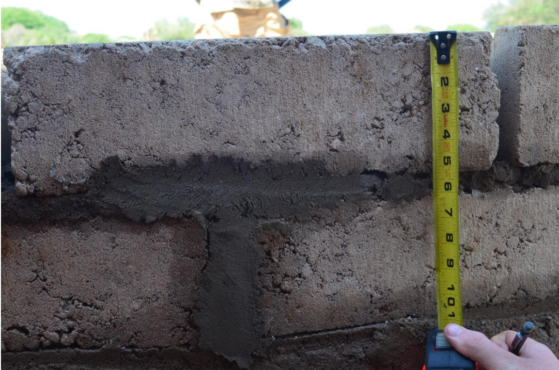
Figure 64: Joint thickness and appearance on outside of tank
