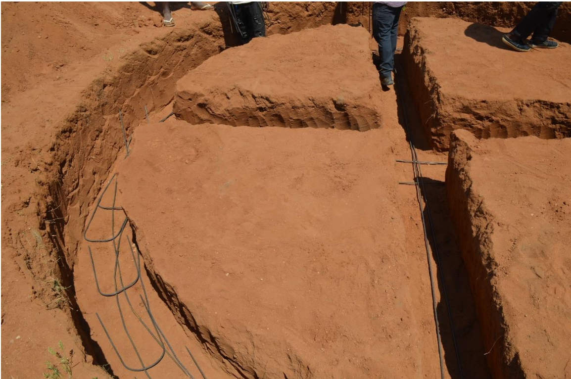
Figure 24: Placing Stirrups underneath Footing Steel
