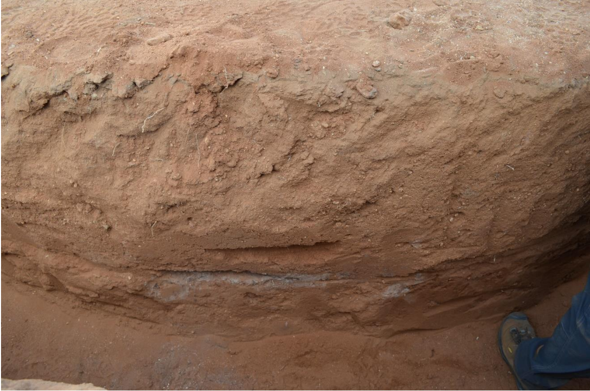
Figure 13: Soil Structure of Footing Excavation
