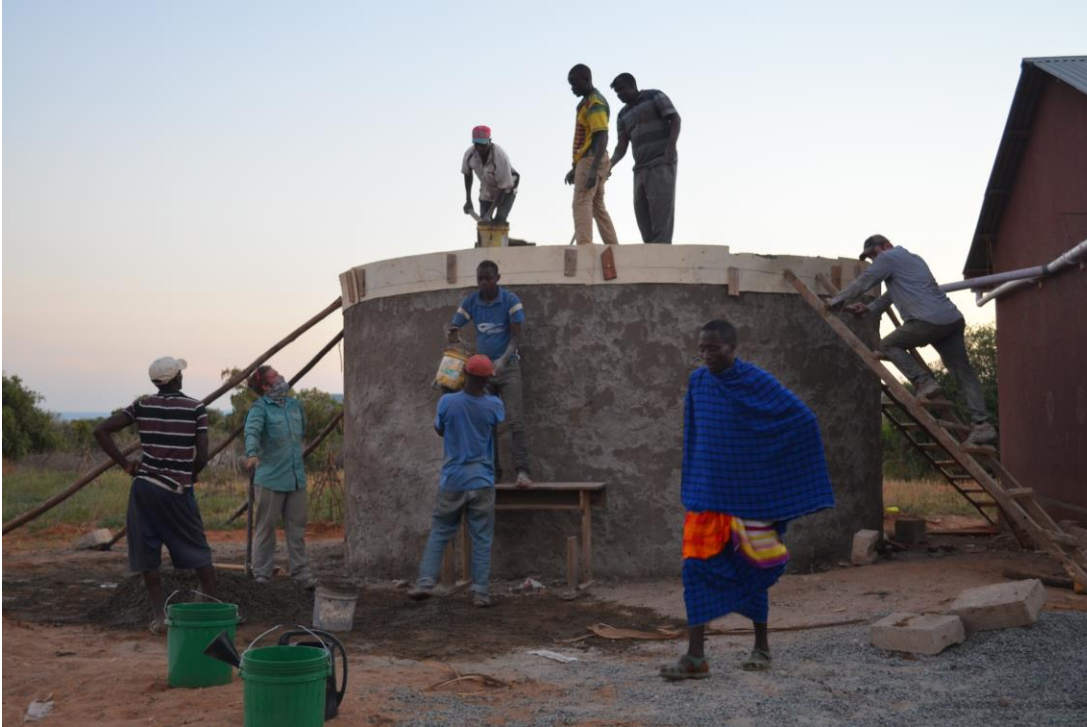
Figure 75: Construction of Top Slab
