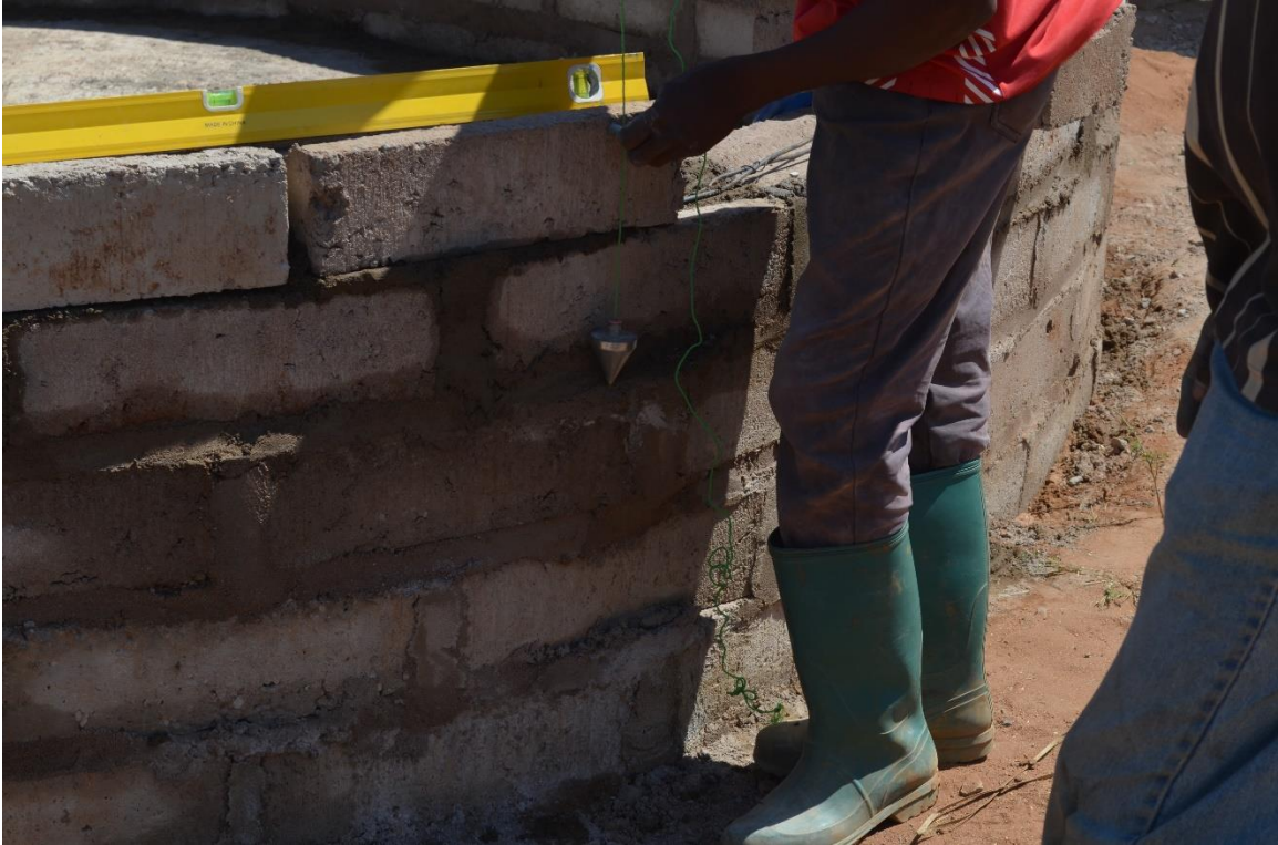
Figure 66: Aligning next course with a plumb bob and leveling course
