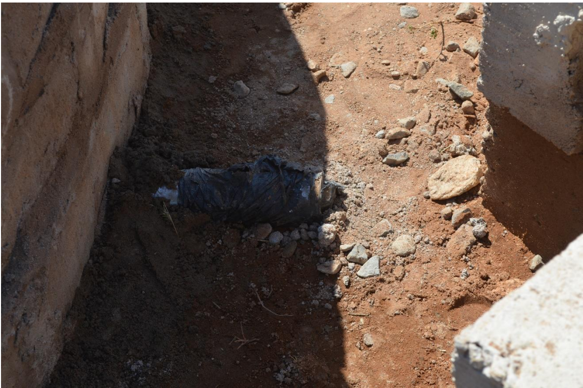
Figure 67: Cleanout location on outside of tank
