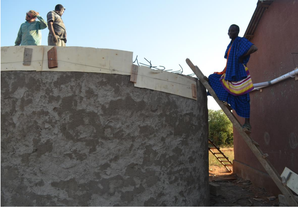
Figure 76: Village Chairmen Inspecting the Top Slab
