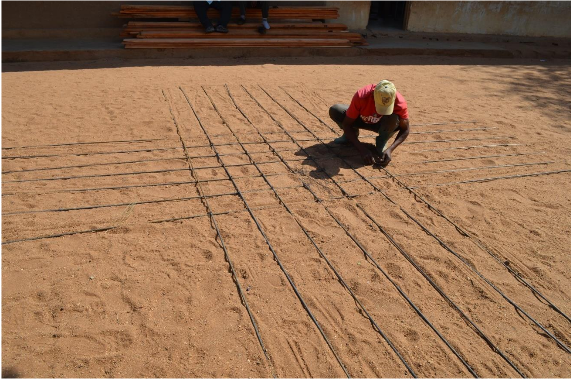
Figure 28: Laying out cut sections for slab steel
