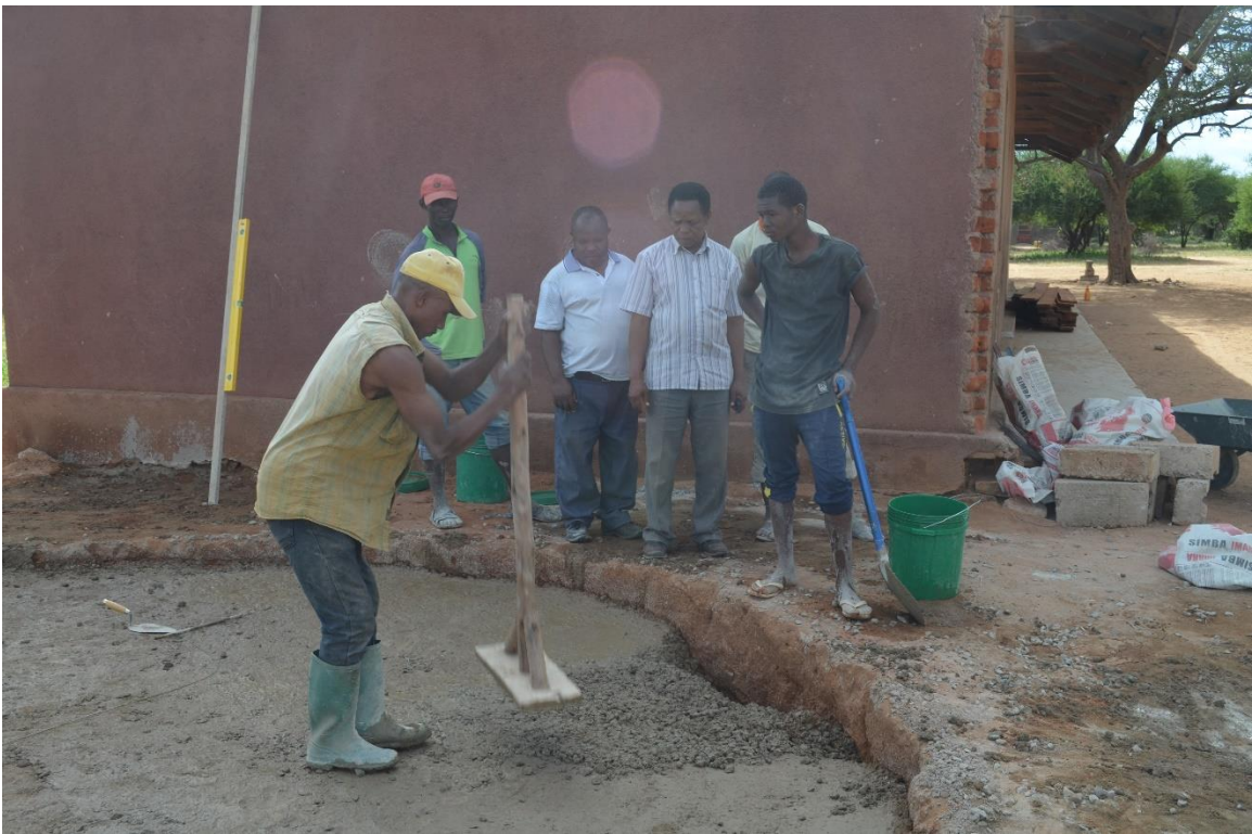
Figure 50: Finishing of foundation slab
