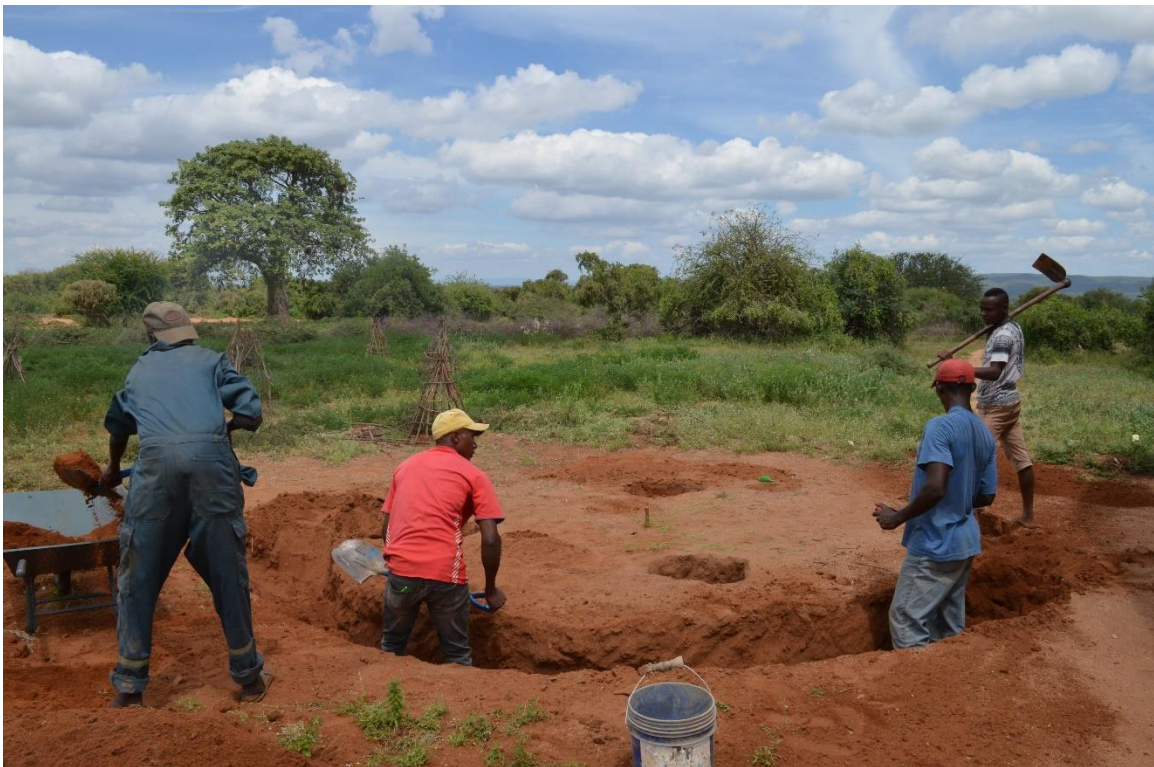
Figure 10: Footing Excavation Continued
