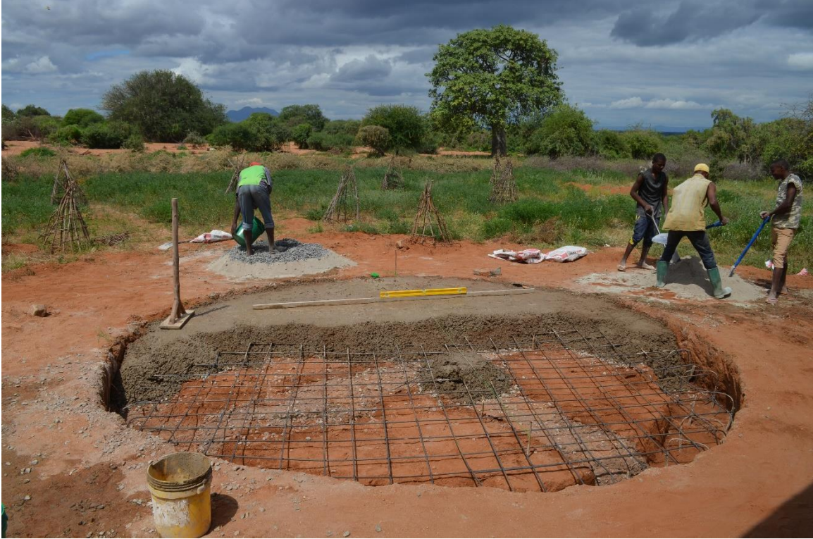
Figure 49: Continuing to place concrete for slab
