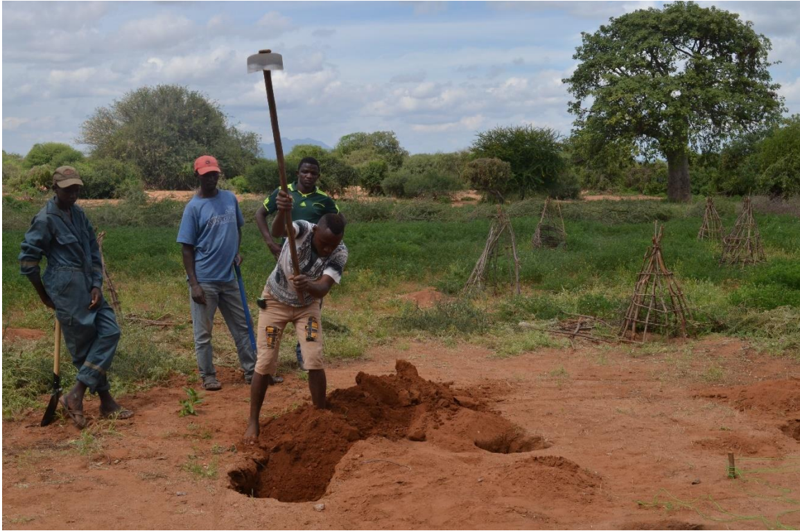
Figure 9: Beginning of Footing Excavation
