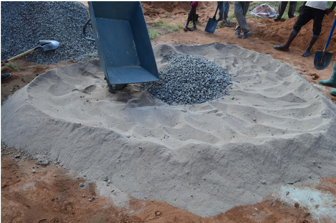
Figure 34: First Batch, using volcano method and adding aggregate into center
