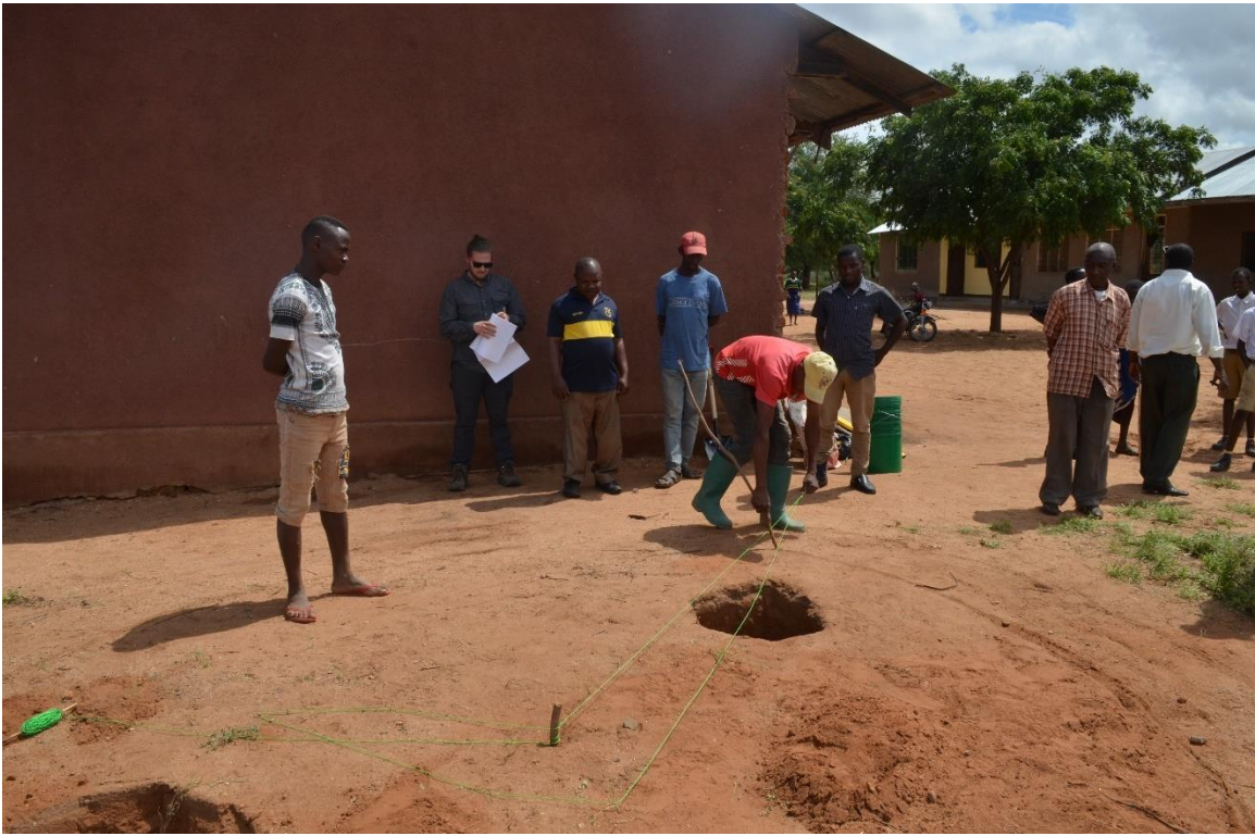
Figure 7: Marking Footing of Foundation 1
