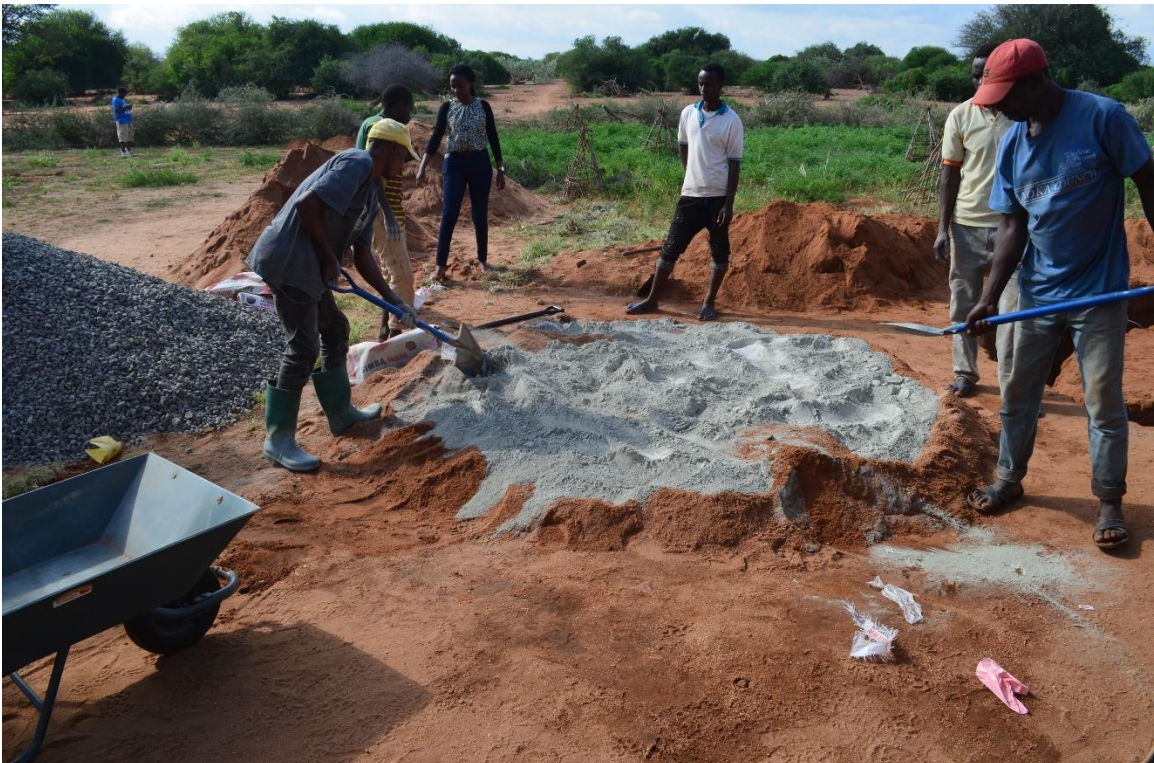
Figure 32: First Batch, Adding cement
