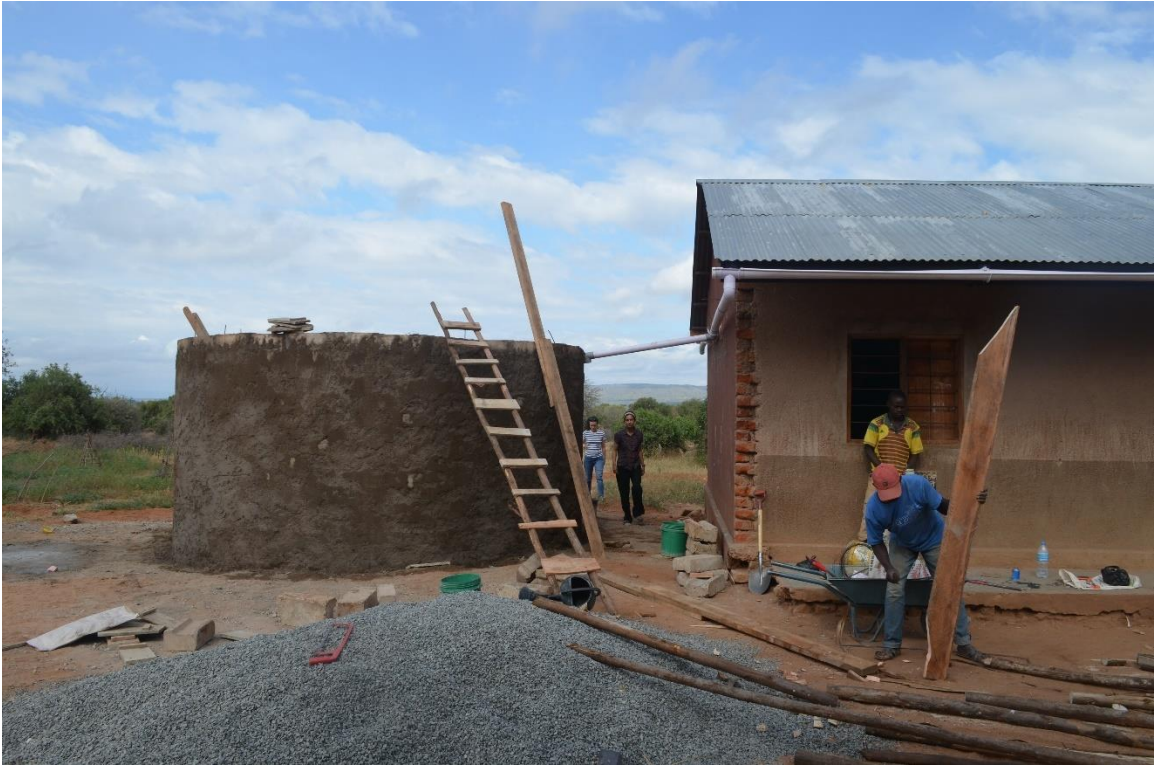
Figure 71: Building the Scaffolding
