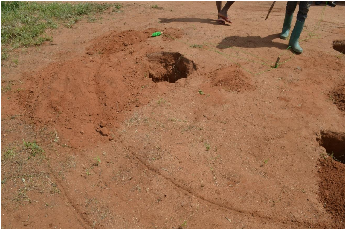
Figure 8: Marking Footin of Foundation 2
