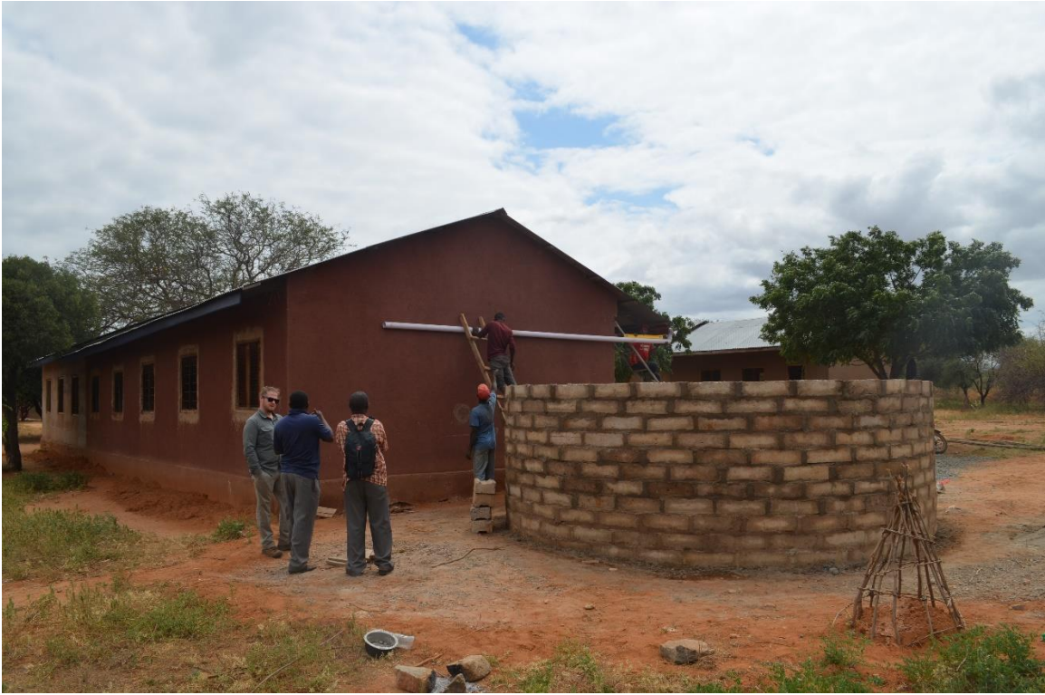
Figure 69: Progression of Wall construction
