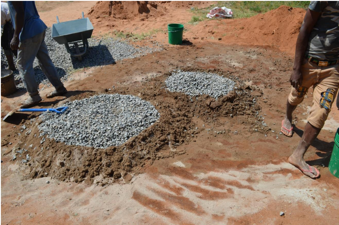
Figure 38: Second Batch, split quantities into two smaller piles
