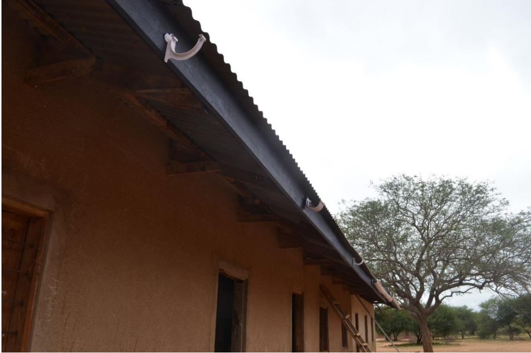
Figure 56: Gutters installed upon arrival on front of school building
