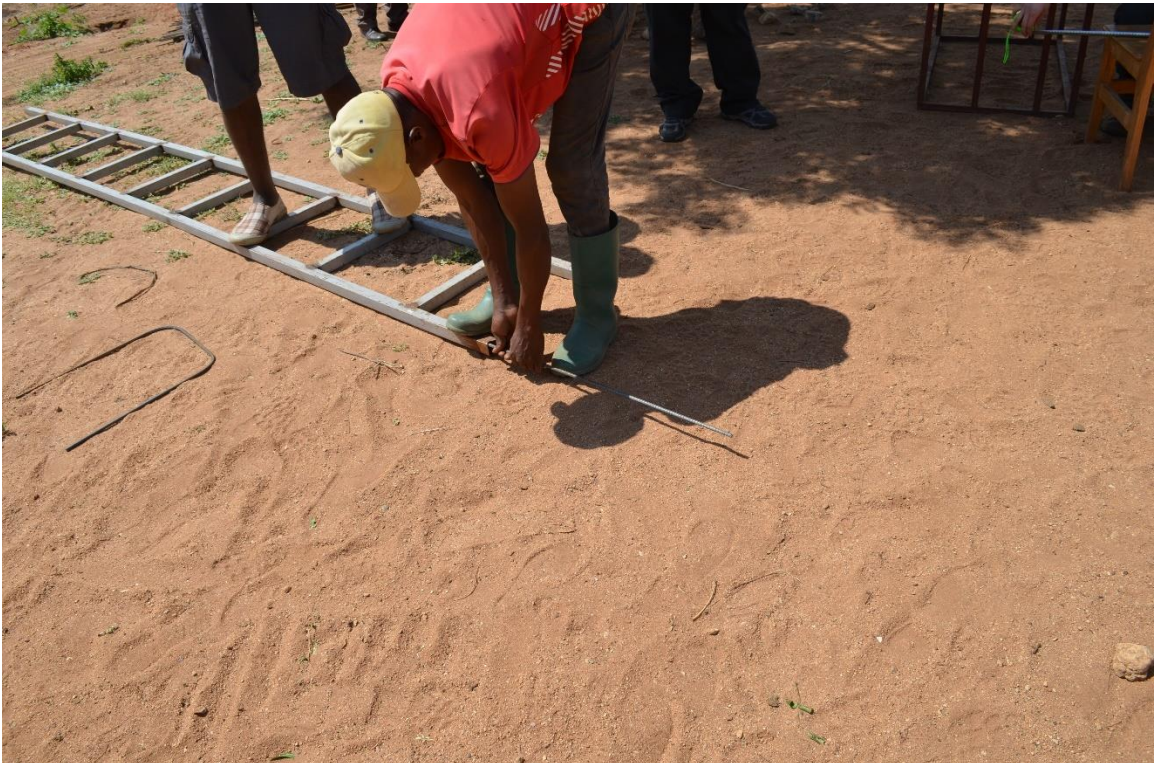
Figure 21: Bending Stirrups using end of a hollow ladder. Trial
