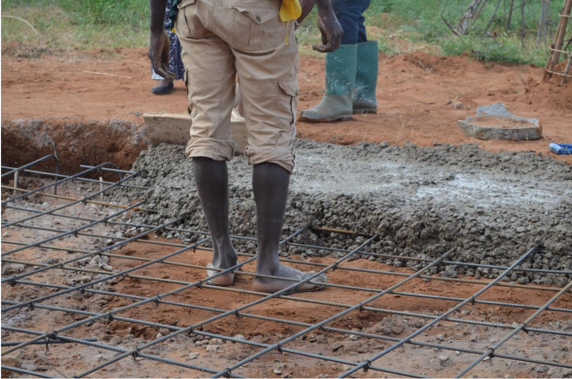
Figure 47: Beginning to place concrete for foundation slab
