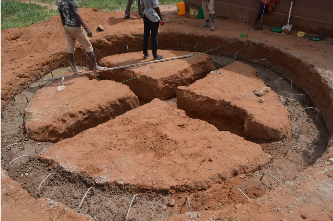
Figure 39: Continuing to place footing
