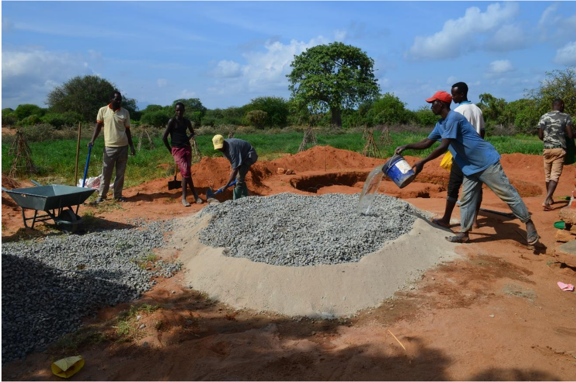
Figure 35: First Batch, Adding water
