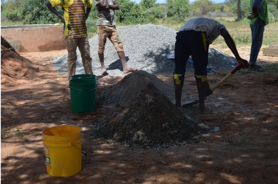
Figure 41: First batch of concrete for blocks (Larger)
