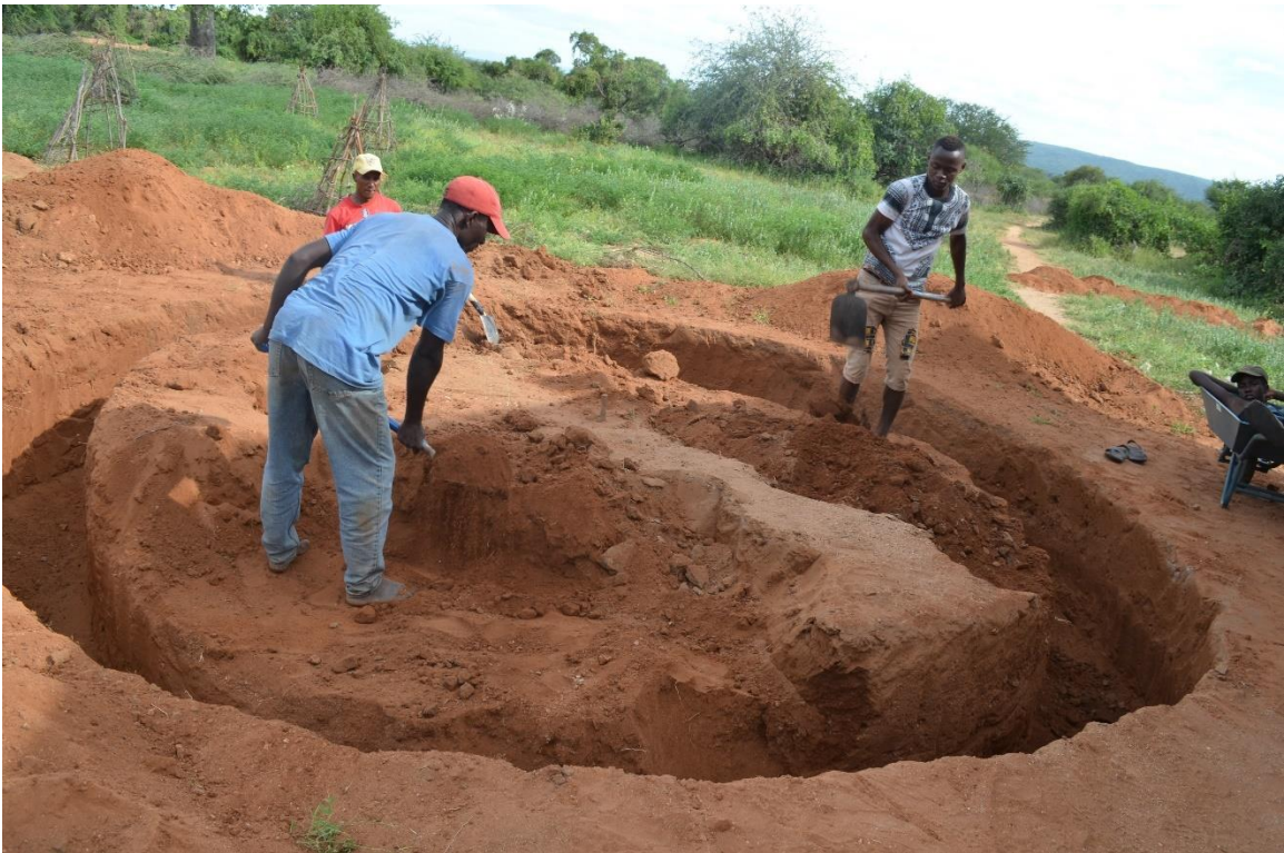
Figure 14: Excavation of Slab Section
