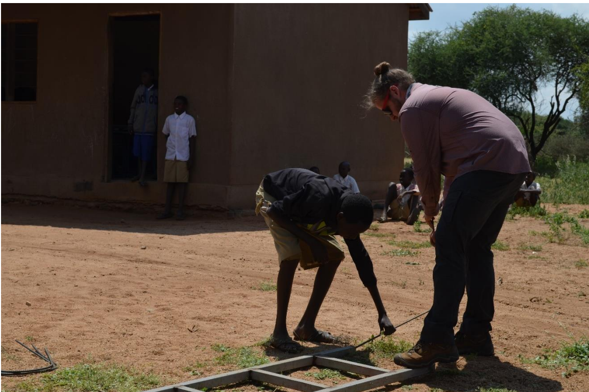
Figure 23: Bending Stirrups based on markings
