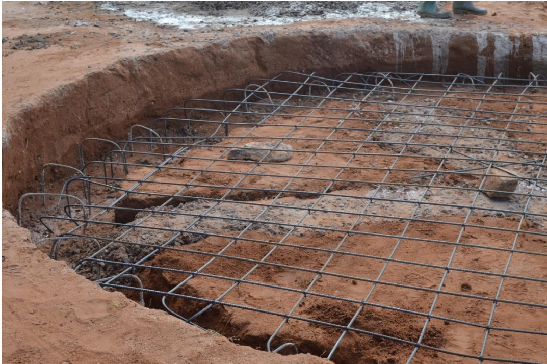
Figure 45: Laying the temperature and shrinkage steel into foundation slab
