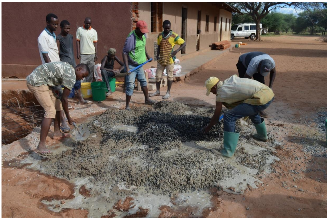
Figure 46: Trying to mix first batch all at one time
