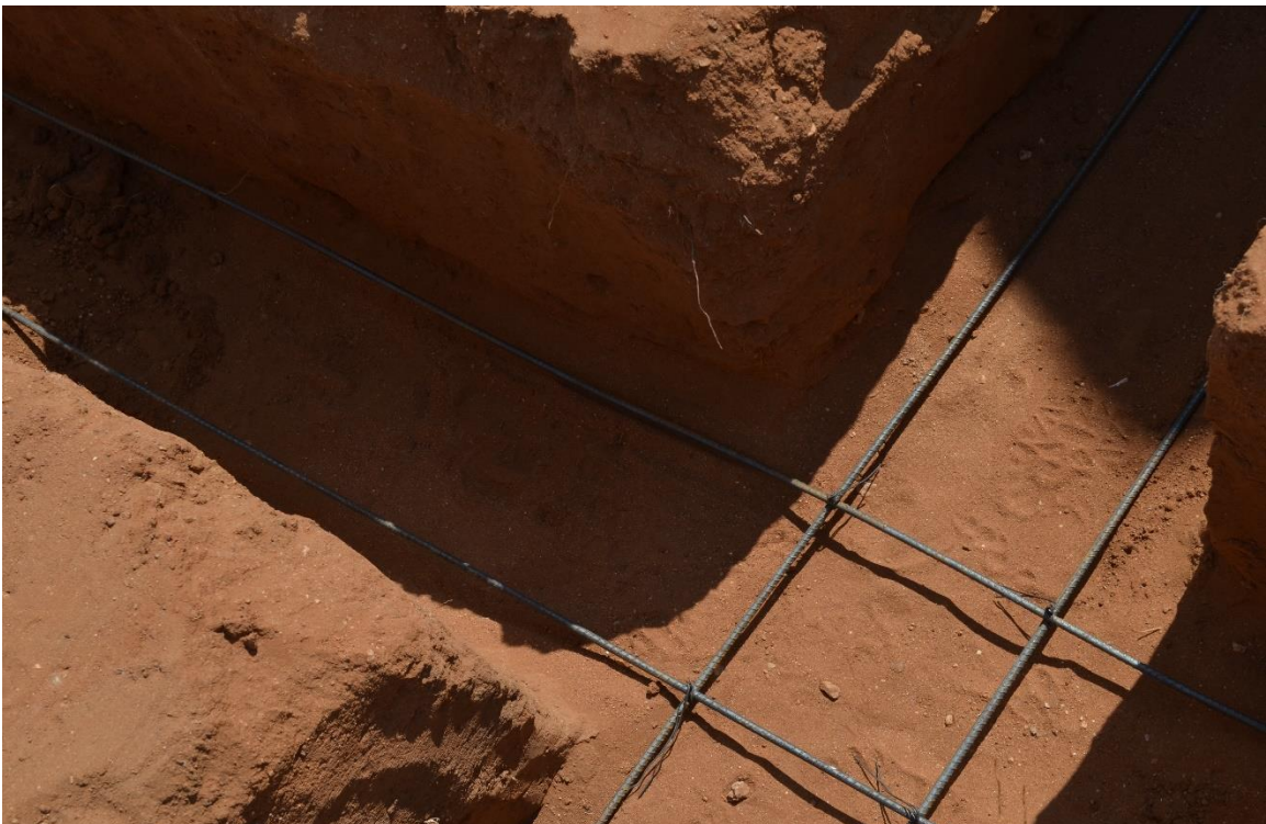
Figure 27: Foundation Beam Steel tied
