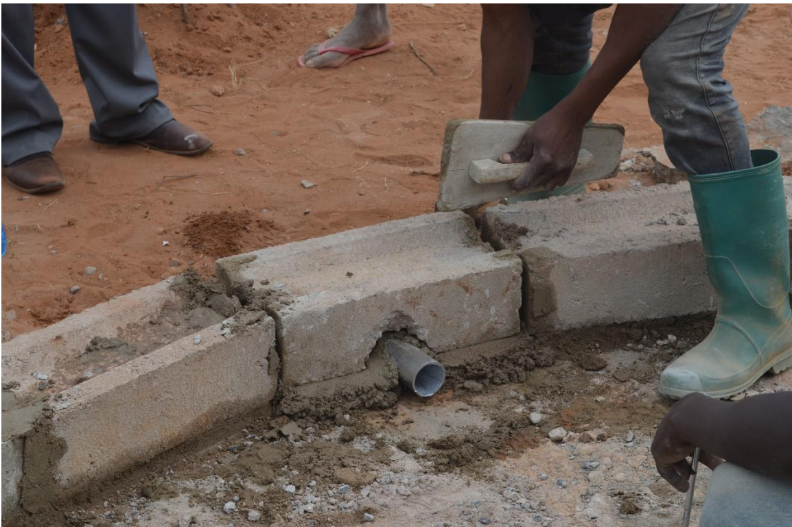
Figure 61: Clean out installment into first course.
