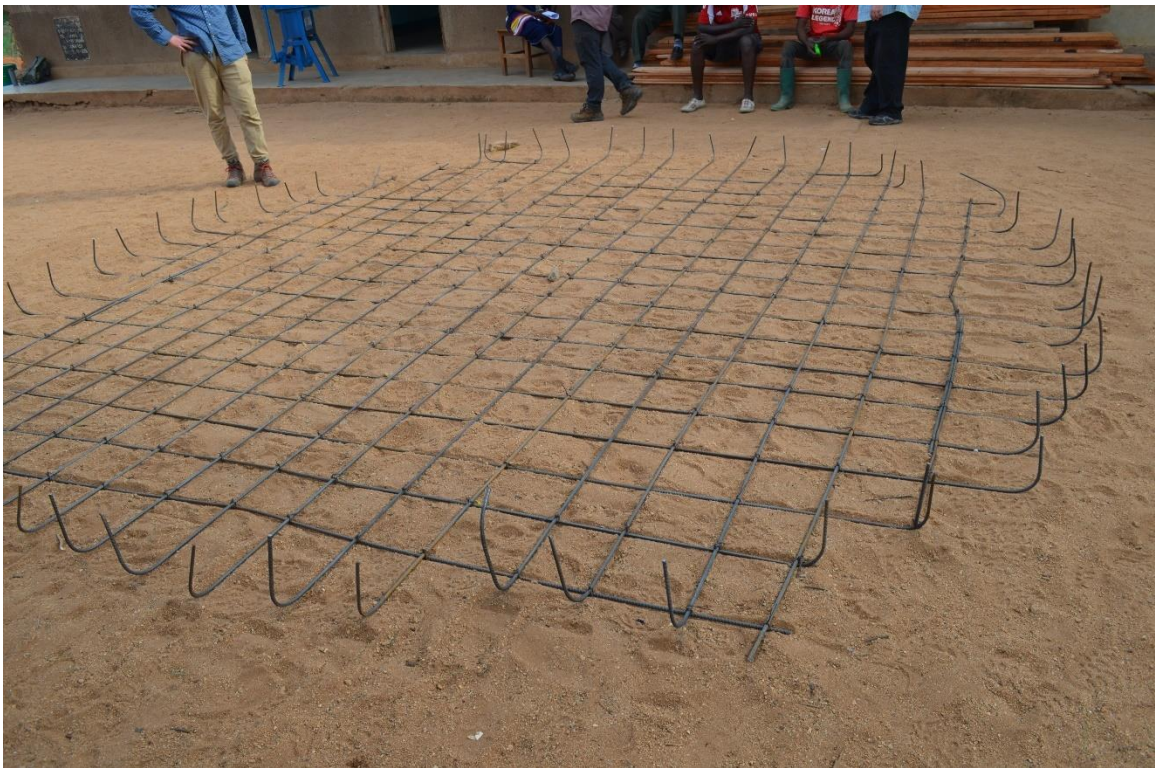
Figure 29: Slab steel tied and bent (upside down)
