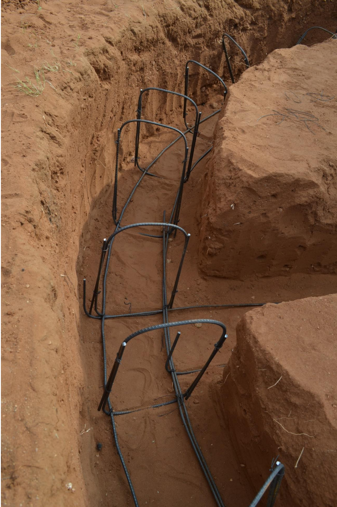
Figure 30: Stirrups completed
