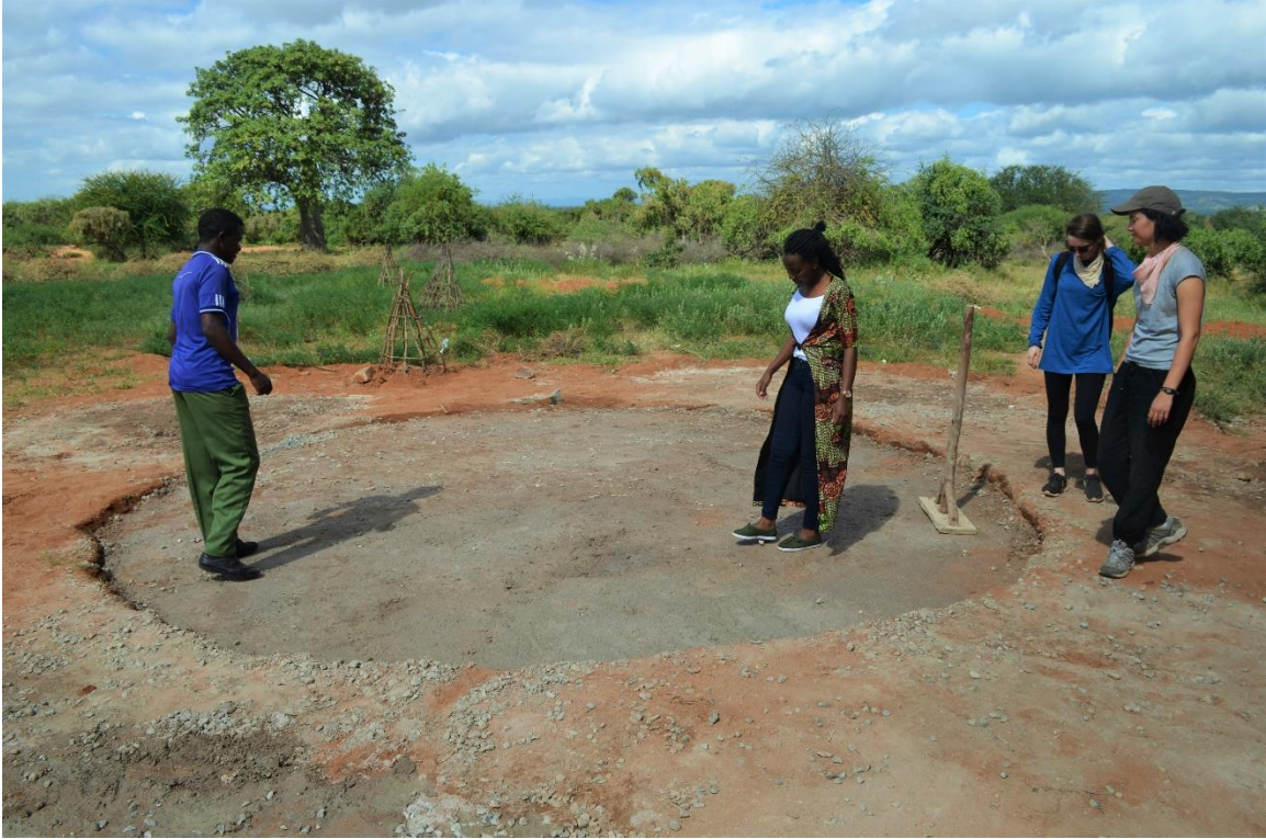
Figure 54: Day after slab placement
