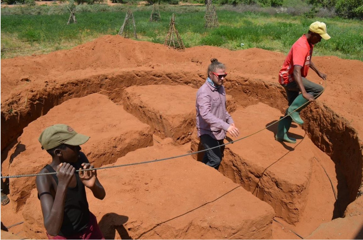
Figure 25: Laying out outside footing rebar
