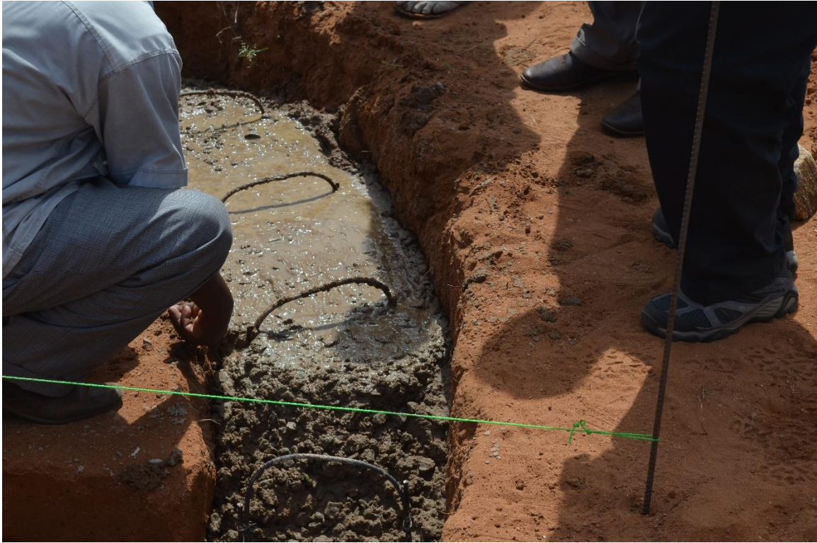
Figure 37: Placing Concrete in Footing
