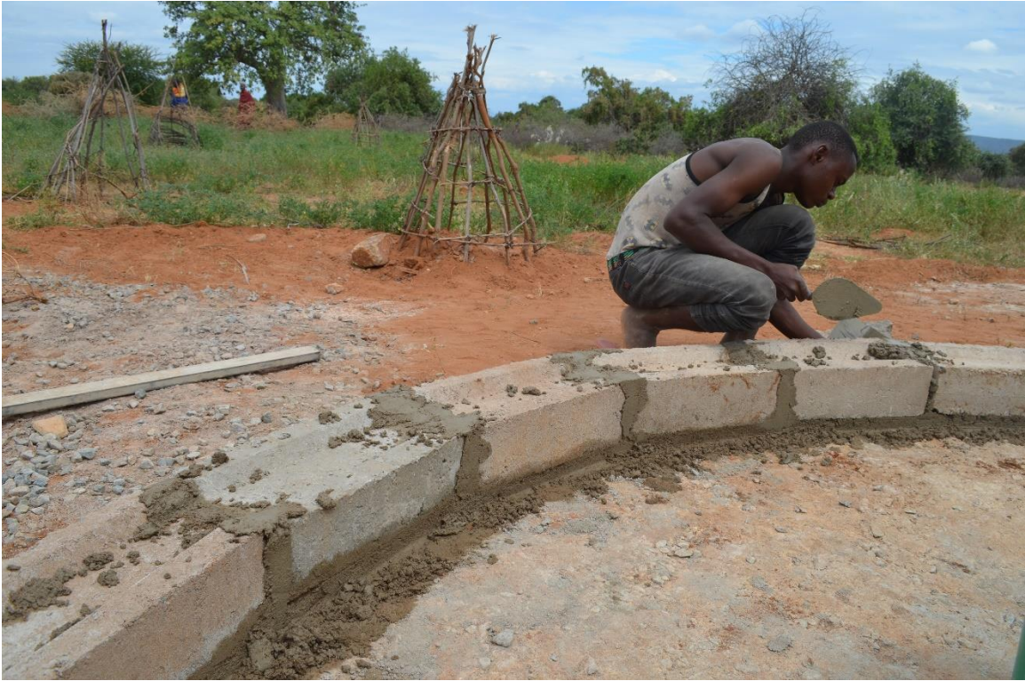
Figure 60: Filling in first course of blocks with mortar.
