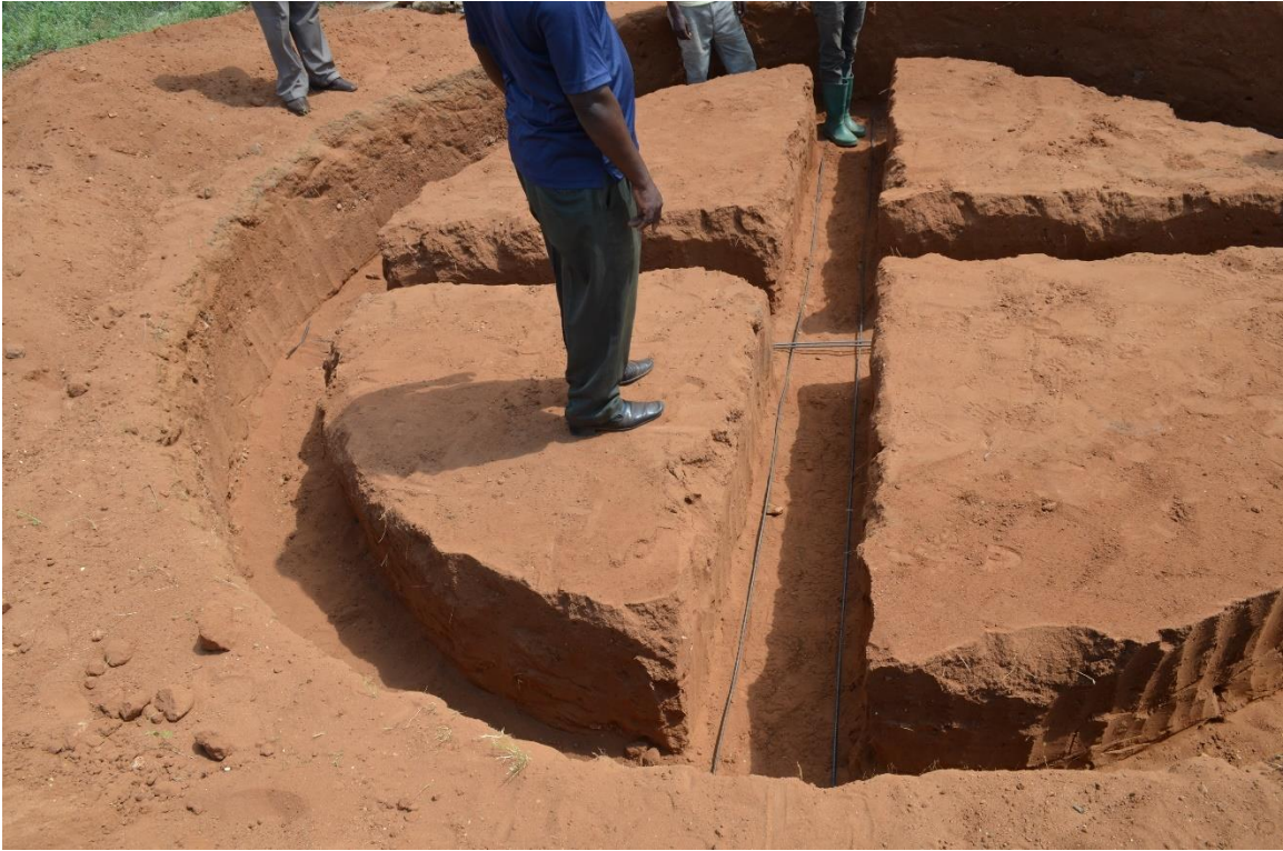
Figure 20: Laying out Beam Rebar
