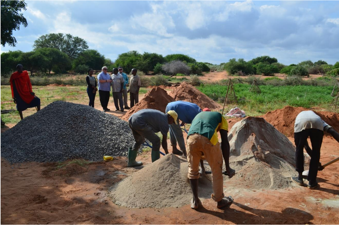
Figure 33: First Batch Mixing Sand and Cement
