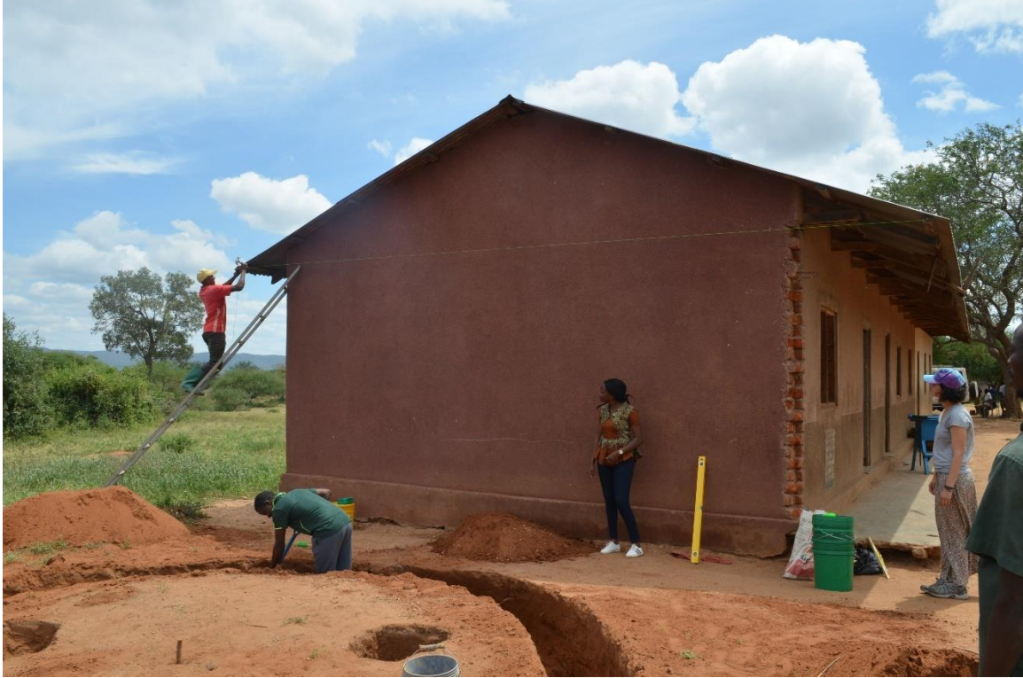
Figure 11: Athumani measuring elevations of roof and foundation
