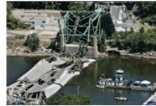
I-35 bridge collapse
