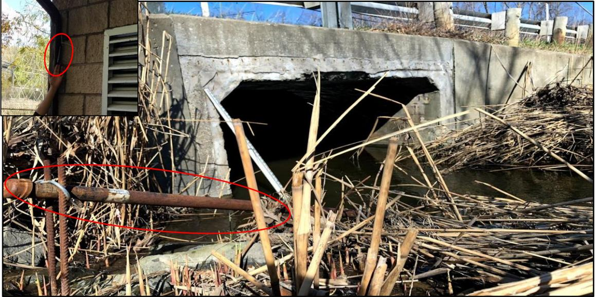
Figure 2-5: Levelogger instrument setup on the upstream side of culvert and Barologger at pump station (top left corner) on Blackbrook road
