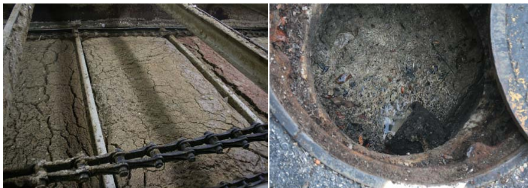
Fig.2.2 (Left) trap grease from Metropolitan Sewer District of Greater Cincinnati; (Right) trap grease from restaurant or residential grease traps
