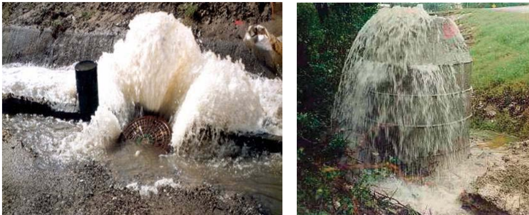
Fig.1.2 Overflowing sewer
