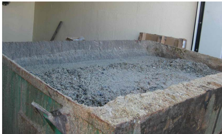
Fig.1.6 Holding tank containing trap grease
