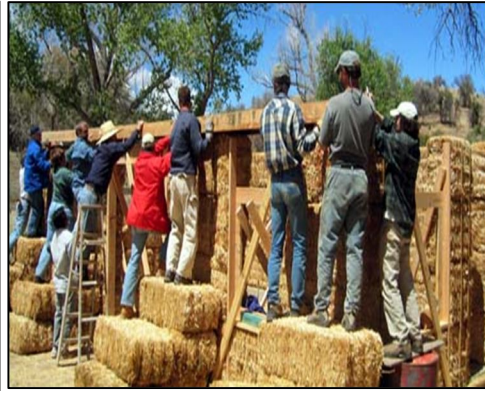
Figure 4.5 Lifting of Roof Plate
