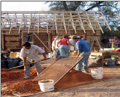
Figure 4.8 Sifting Plaster Mix
