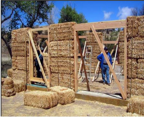
Figure 4.4 Bale Wall System
