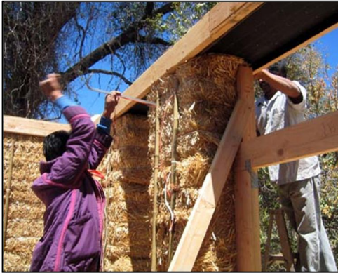
Figure 4.6 Fastening and Tie Ins
