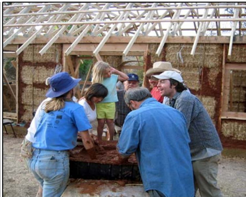
Figure 4.9 Mixing Lime and Clay Rendering
