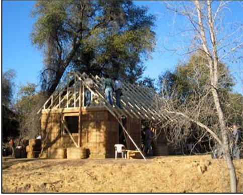
Figure 4.10 House Prior to Plastering
