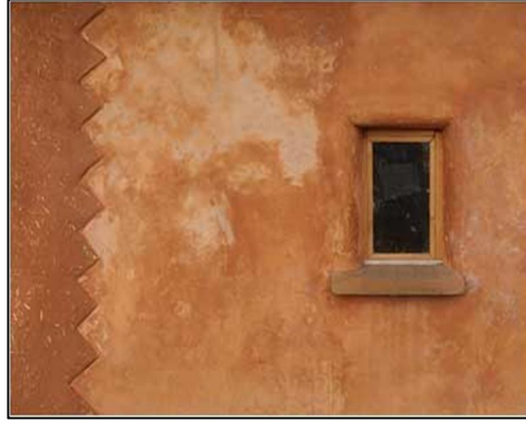
Figure 4.11 Finished Clay Rendering
