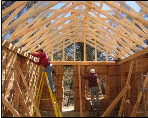
Figure 4.7 Roof Truss
