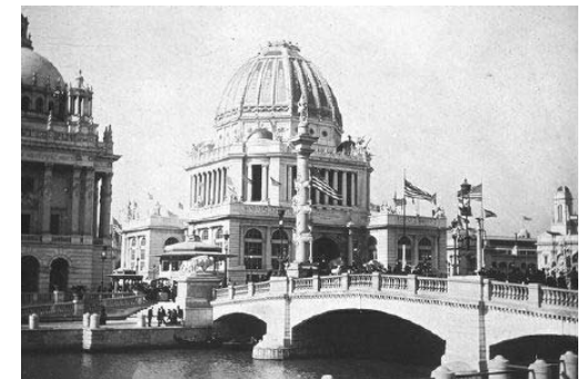
Figure 1.10 Administration Building at Chicago Exposition
