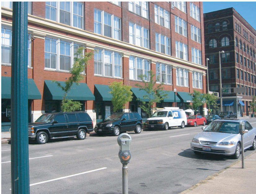
Context: View looking East on Eighth Street to the renovated Power Building Apartments
