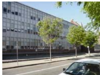
Figure 3.11 Washington Park Elementary School located in inner-city Cincinnati, Ohio
