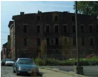
Figure 5.8 Over-the-Rhine – downtown Cincinnati, Ohio – dilapidated building's are the norm
