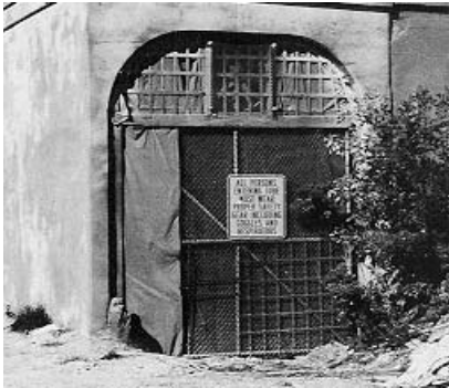
Figure 5.3 Cincinnati Subway – closed tunnel – a daily reminder
