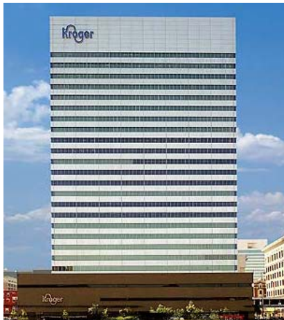
Figure 5.10 Cincinnati, Ohio – Kroger Corporation's Corporate Headquarters, located downtown – employee parking garage to be built across the street, at the city's expense
