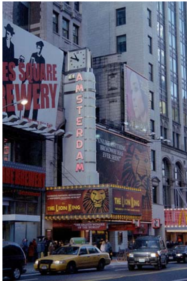
Figure 3.30 Renovated Amsterdam Theater – New York City
