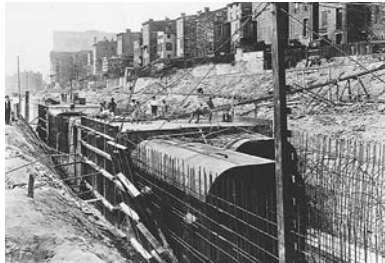
Figure 3.16 Cincinnati Subway – under construction circa 1924
