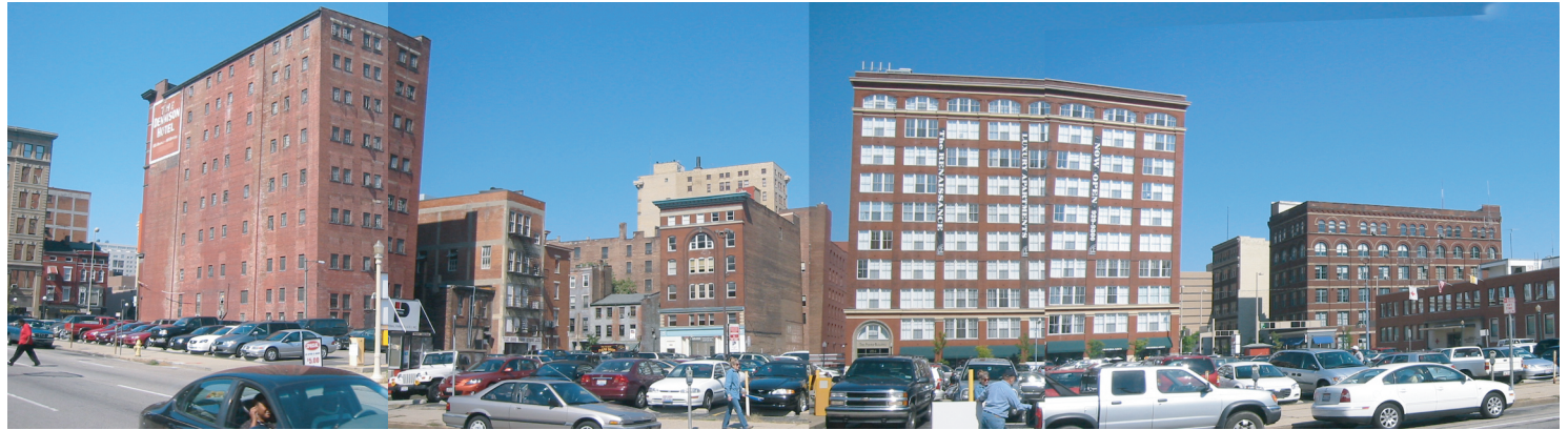
Project Site - View looking North to existing surface parking lot - Dennison Hotel is to the left of the image
