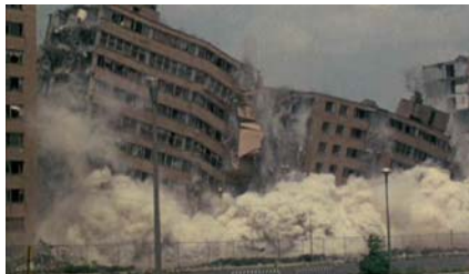
Figure 2.21 Pruitt Igoe – St. Louis, Missouri – demolition, 1972
