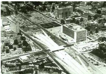
Figure 2.17 The same community during the Urban Renewal program...
