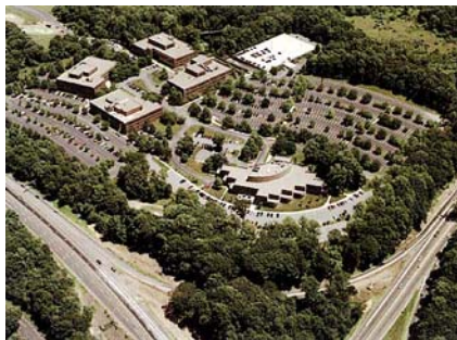
Figure 2.25 Suburban Office Park – aerial view
