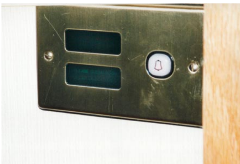
Fig. 3.15 The picture to the right shows a panel located at the bedside table. The two buttons (Don Not disturb, and Please Clean Room) if pressed, will turn on the indicators located outside the guestroom door (shown on the picture to the left). Source: personal photography at the Crowne Plaza Dubai.
