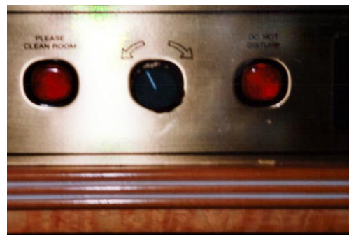
Fig. 3.15 The picture to the right shows a panel located at the bedside table. The two buttons (Don Not disturb, and Please Clean Room) if pressed, will turn on the indicators located outside the guestroom door (shown on the picture to the left). Source: personal photography at the Crowne Plaza Dubai.
