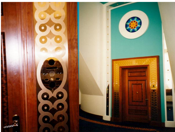
Fig. 4.24 Surveillance camera and entry system is located at each guestroom entry.
