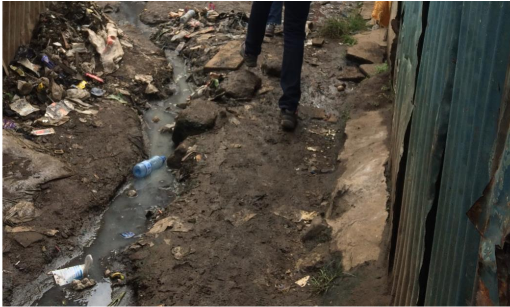
Figure 7: Divert carved into a walkway to prevent water from getting in the homes
