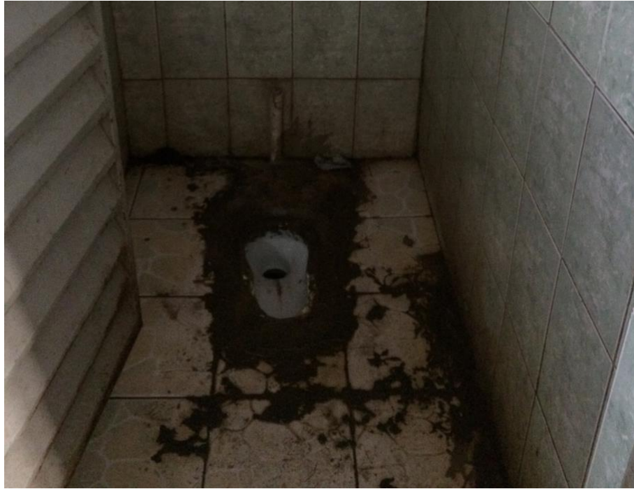
Figure 2: Pour-flush toilet in a public toilet stall in Mathare
