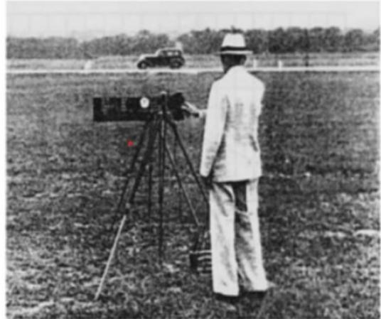
Figure 2.1: Traffic theory in the 1930s: Historical speed-density diagram and the experiment carried out by Bruce D. Greenshields. [From Greenshields, B.D., A study of traffic capacity. In: Proceedings of the Highway Research Board, Vol. 14. Highway Research Board, Washington, D.C. (1935)]
