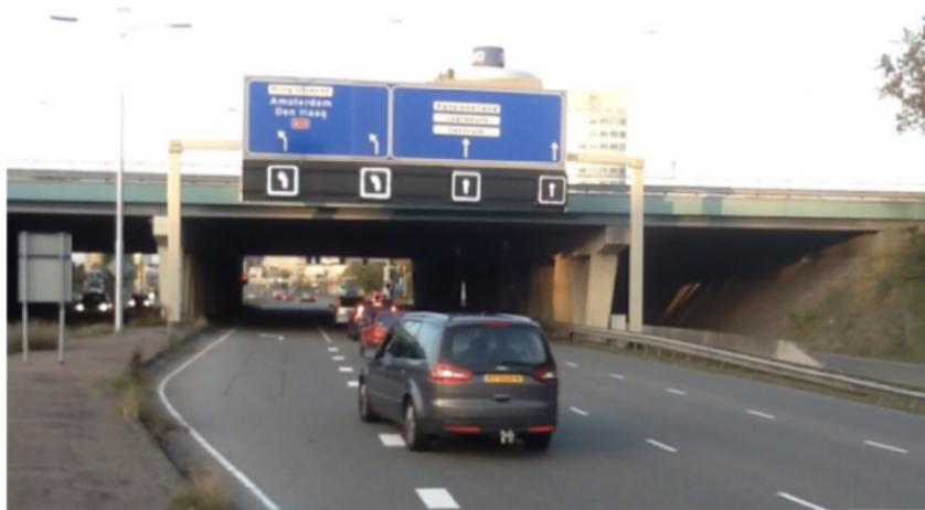
Figure 7.1: Dynamic message signs indicate the lane use at the intersection in Utrecht, The Netherlands(Courtesy of Anema(2015))
