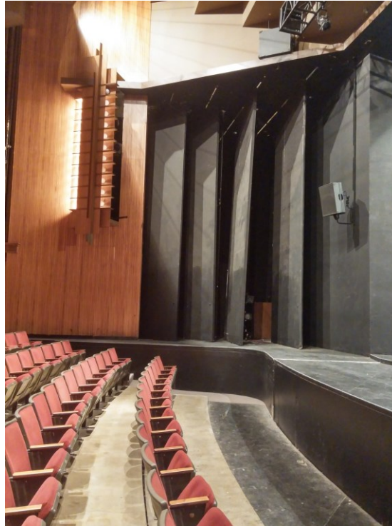
Figure 2. Stage Right Wing with Caliper Doors and partial Orchestra Pit Lift
