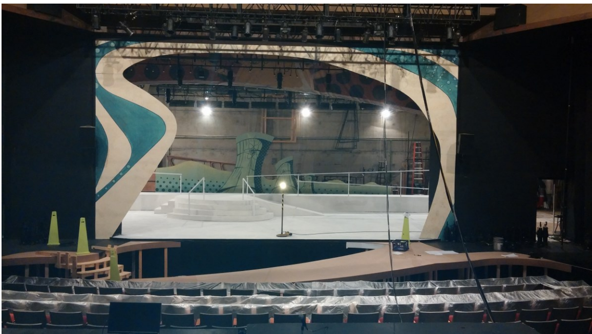
Figure 33. Process Shot of the Finished Floor and Base Coat of Paint Laid.
