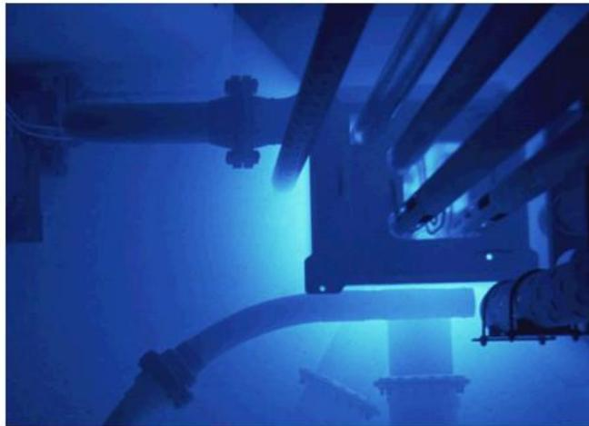
Figure 13: The open pool research reactor at The Ohio State University. The blue glow comes from Cherenkov radiation in water.
