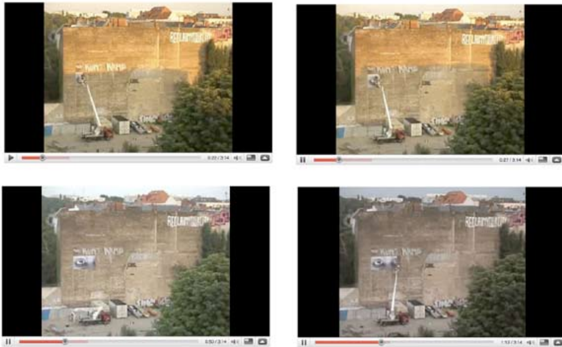
Figure 4.2. Installation process of JR
