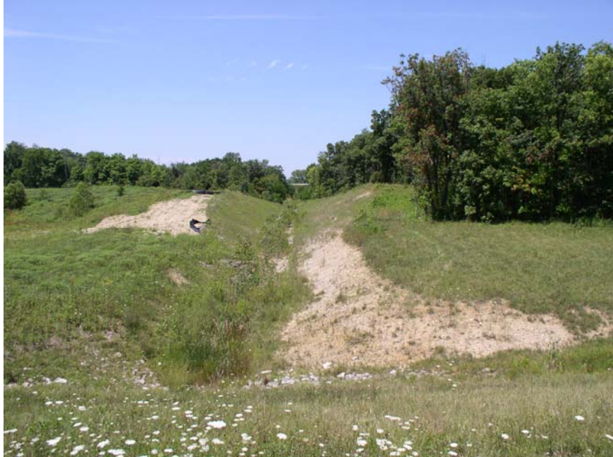
Figure 4.3: Logan County 33/347 drainage channel (facing NE), August 2004.
