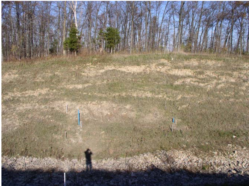
Figure 4.6: Scarps and erosion on the northeast slope, November 2005.
