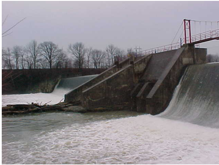
Figure 1.2: Downstream view of the Ballville Dam
