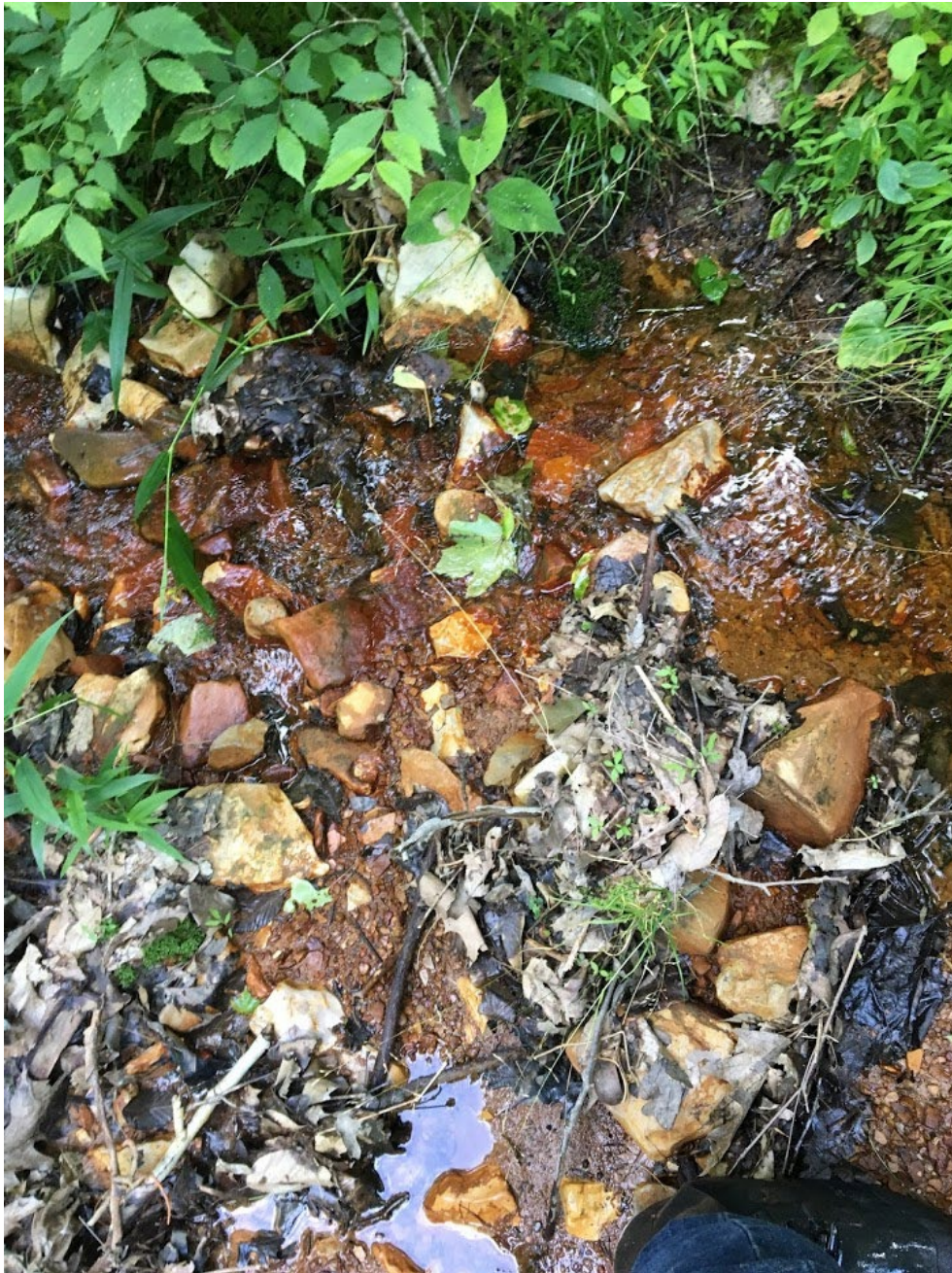
Figure 60 Orange colored precipitate of stream bed at Sines No. 2 discharge. This is likely precipitated iron hydroxide (yellowboy).
