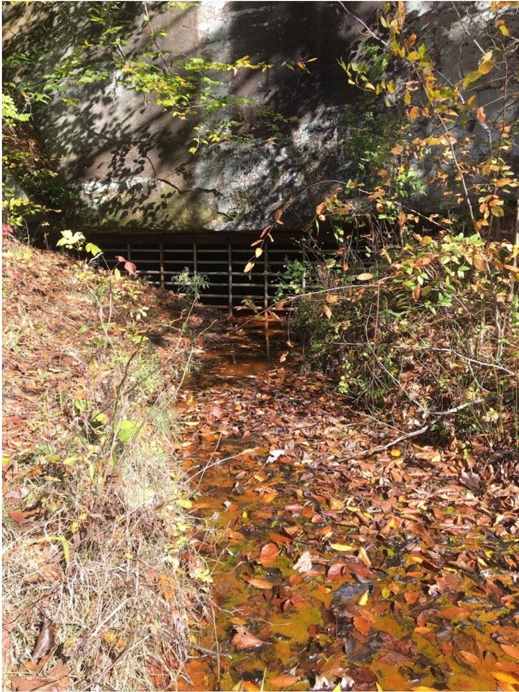
Figure 61 Yellow and orange colored mineral precipitate thickly coating stream bed of the Pine Run (Sunday Creek No. 9 and 12) mine effluent creating a false bottom. This is likely a large portion of iron hydroxide (yellowboy) deposition from accumulated forms of iron hydroxide.
