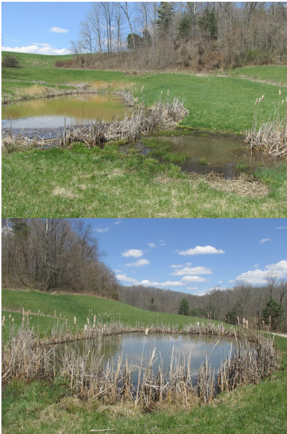
Figure 14. Photographs of the constructed wetland cell 2 and limestone drain (top), and cell 3 (bottom).
