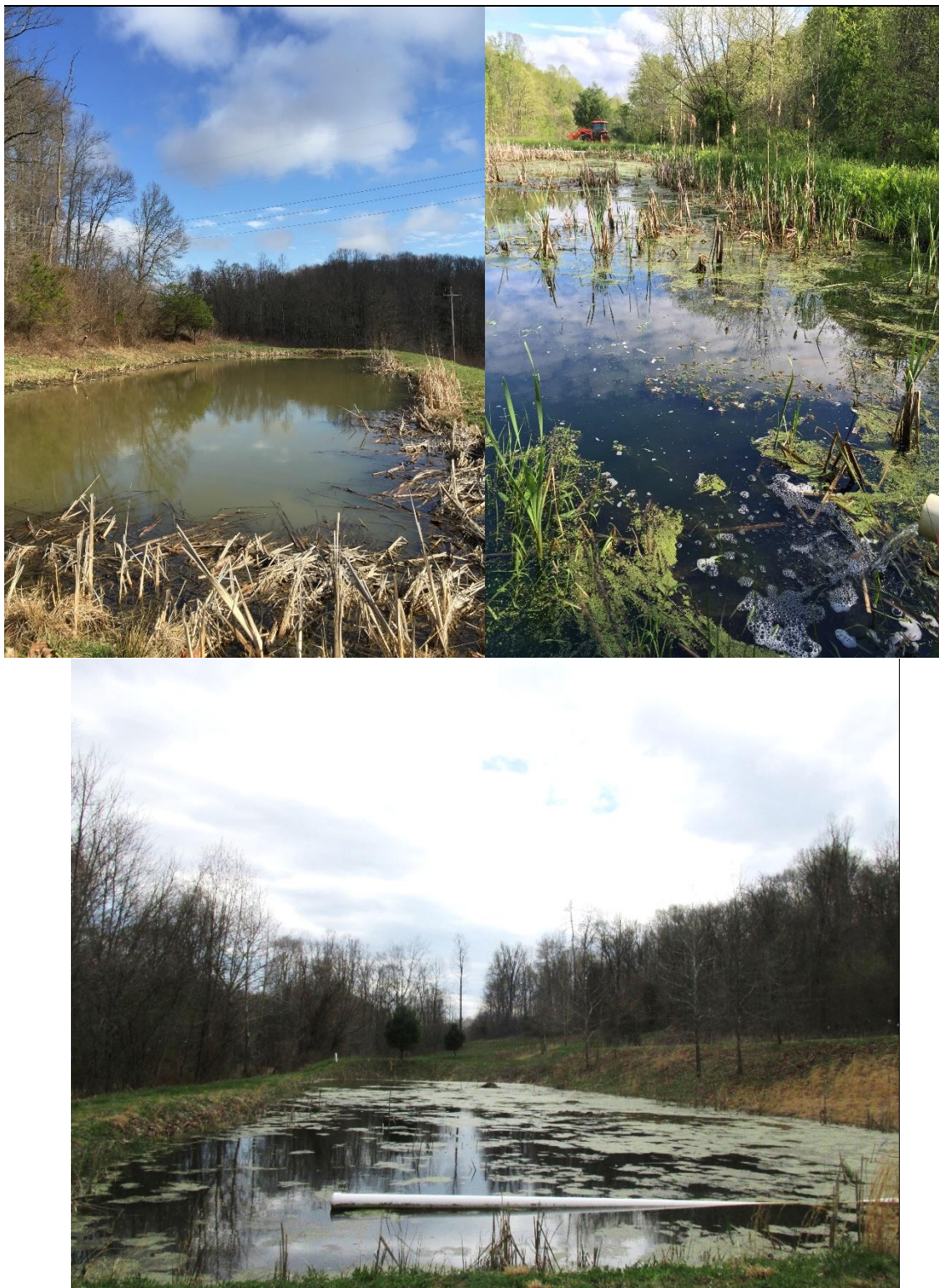
Figure 15. Photographs of the constructed wetland cell 4 (top-left), cell 5 (top-right), and cell 6 (bottom).
