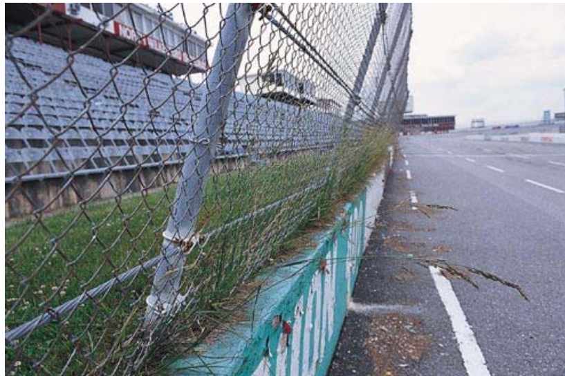
Figure 3.6: Grass is starting to grow through the fences and over the track's walls.
