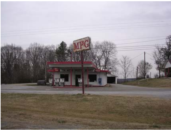
Figure 4.7: This closed-down service station is located at the intersection of U.S. Highway 421 and Speedway Road.
