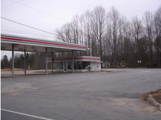
Figure 4.5: A modern service station along Speedway Road that is no longer operating.
