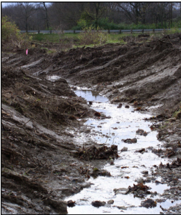
Figure 3. Existing Stream has been graded and left undisturbed
