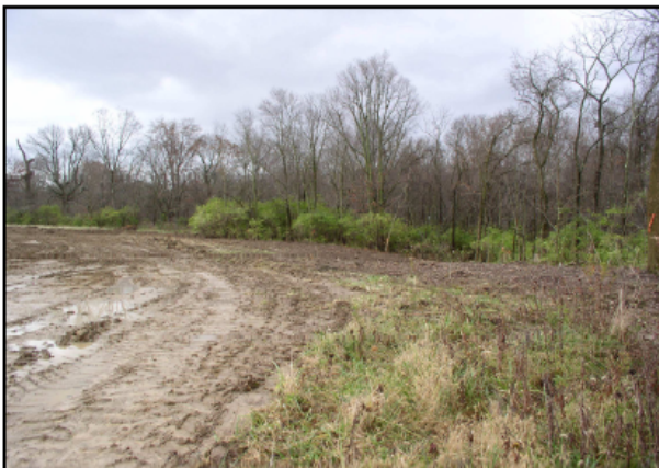
Figure 5 Northeast Lots need perimeter controls (silt fence or mulch berms)
