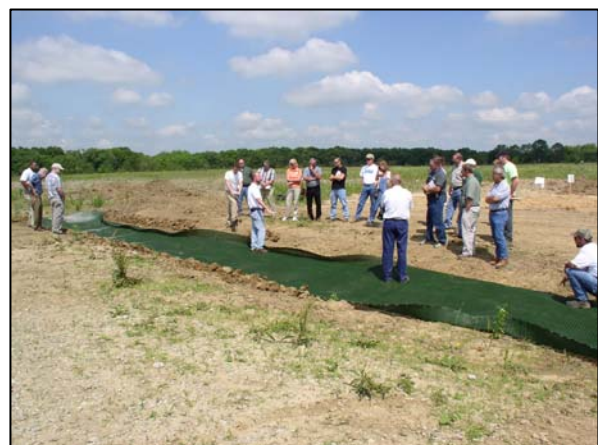
Figure 17. Demonstration of Erosion Control Matting
