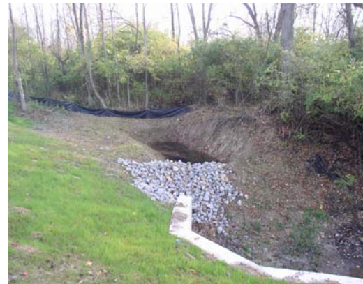
Figure 6. Silt trap serving as stream protection (Rentschler Estates)
