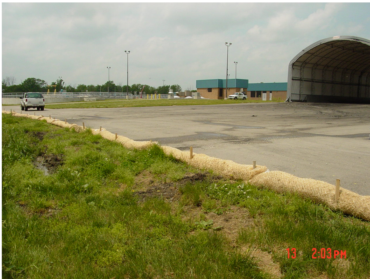
Figure D: Sediment logs placed around the biosolids storage area at Upper Mill Creek WRF as part of the SWPPP
