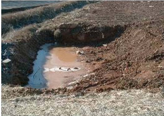
Sediment traps are used to collect sediment-laden runoff from disturbed areas on construction sites
