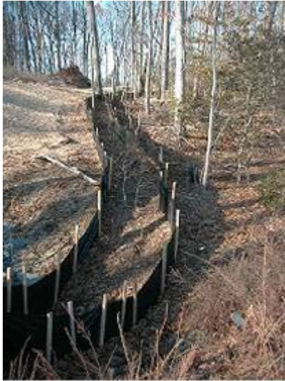
Silt fences prevent the offsite transport of sediment
