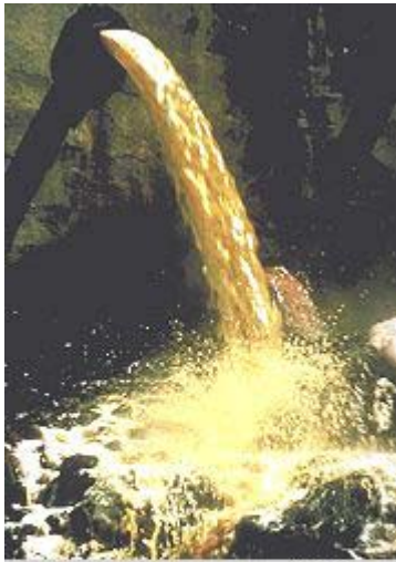
Municipalities can establish a program to inspect storm drain systems for connections to the sanitary sewer system to prevent discharge of untreated wastewater to waterbodies
