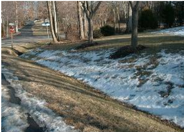
A grass-lined channel can be used to filter and convey runoff
