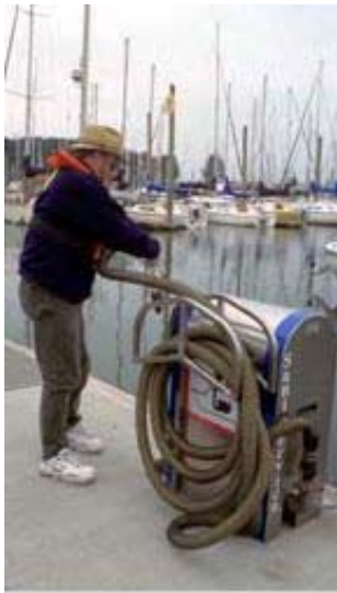
Many marinas provide pumpout stations for safe disposal of bilge (Source: Oregon State Marine Board, no date)
