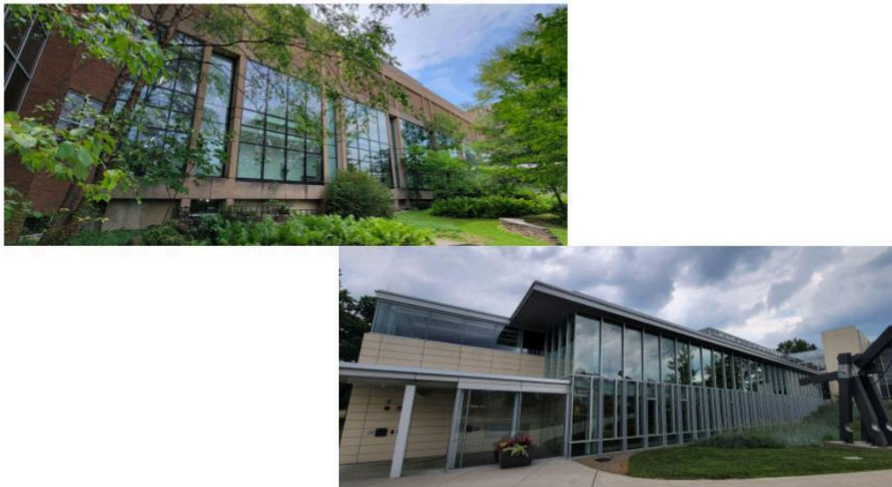
Figure 9. Top Image: Back-side of Cunningham Hall– an example of dense vegetation surrounding areas of windows and near the ground. Bottom Image: Side of DI Hub– example of little to no vegetation. Additionally, the DI Hub was the only building surveyed that had a fritted pattern in the windows to prevent collisions on the Kent State University campus.
