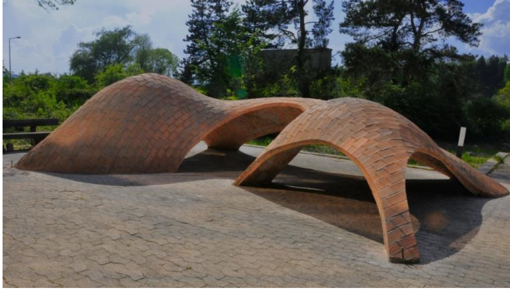
Figure 2.14: Examples of free-form masonry shells (a) Free-form brick structure by ADAPt, Iran (image: Mohammad Soroosh Jooshesh www.archdaily.com ) (b) Free-form tile vault, Zurich, Switzerland, 2010 (image: Klemen Breitfuss)
