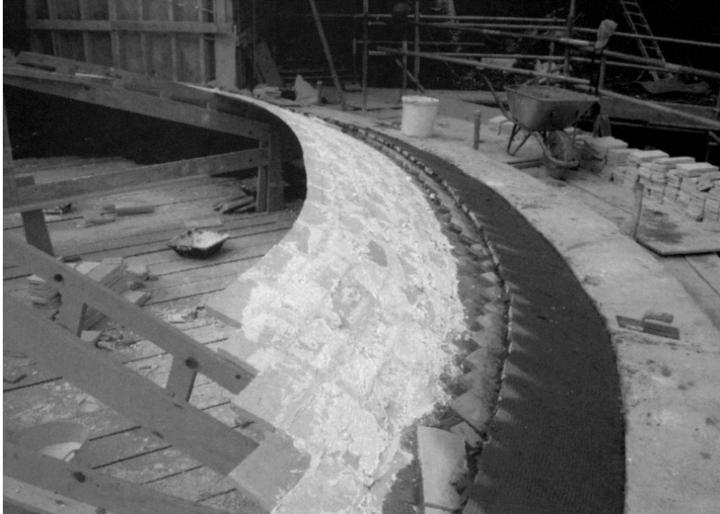
Figure 2.22: Tile Layering technique in Guastavino construction (Ramage, 2007)
