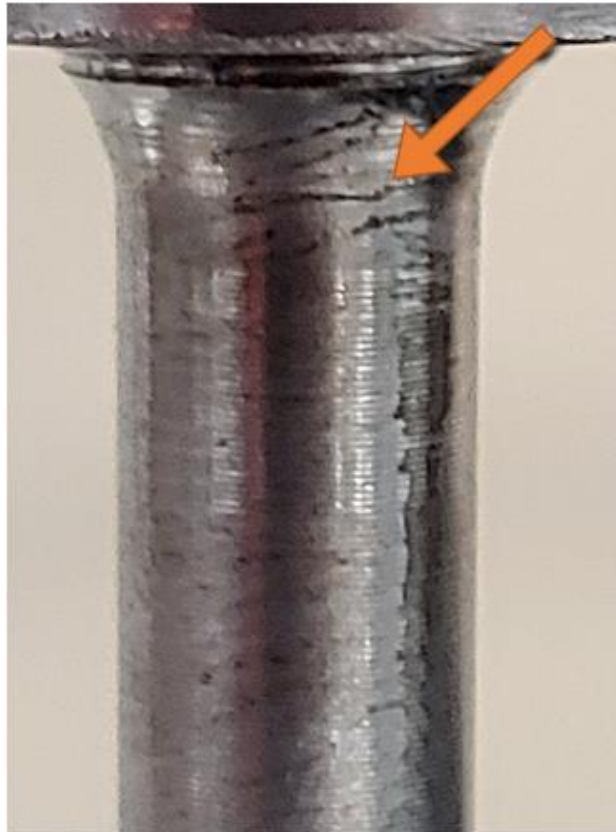
Figure 21: Visible Cracking in the Transition Radius of unfocused beam, heat treated specimen
