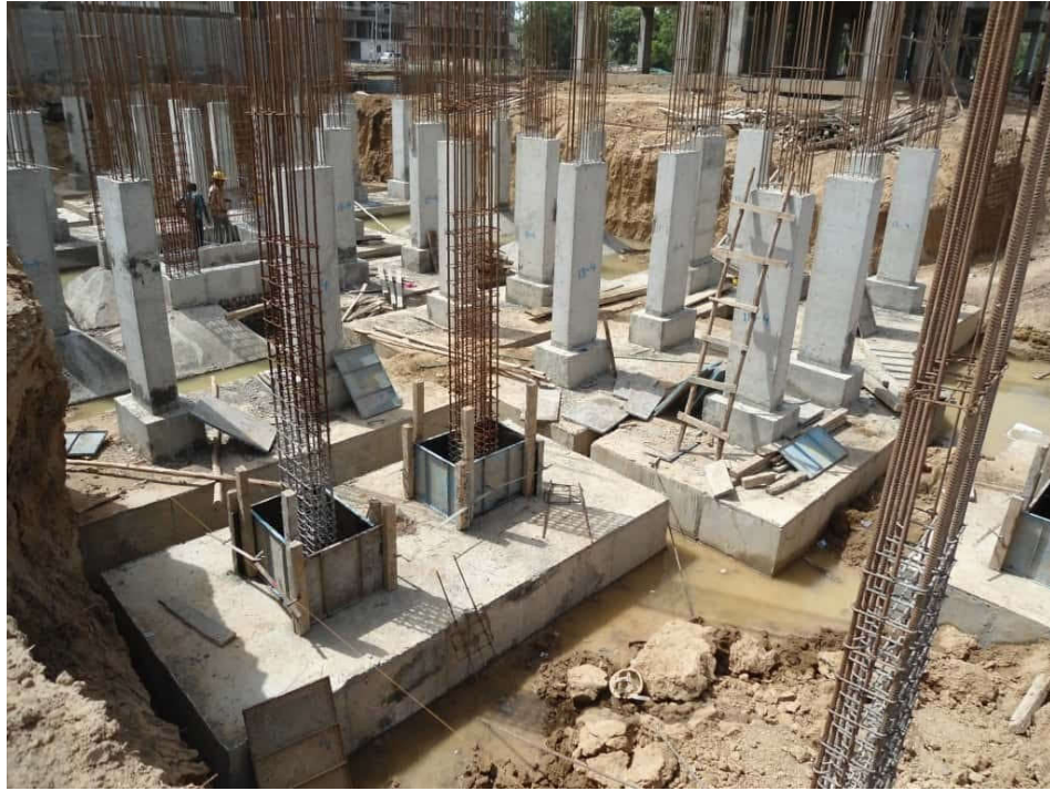
Figure 1. Rectangular combined footings [7].
