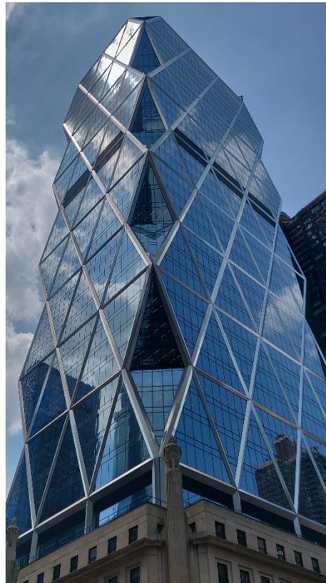
Figure 6.2 Hearst Tower, New York City, one the first iconic steel diagrid buildings
