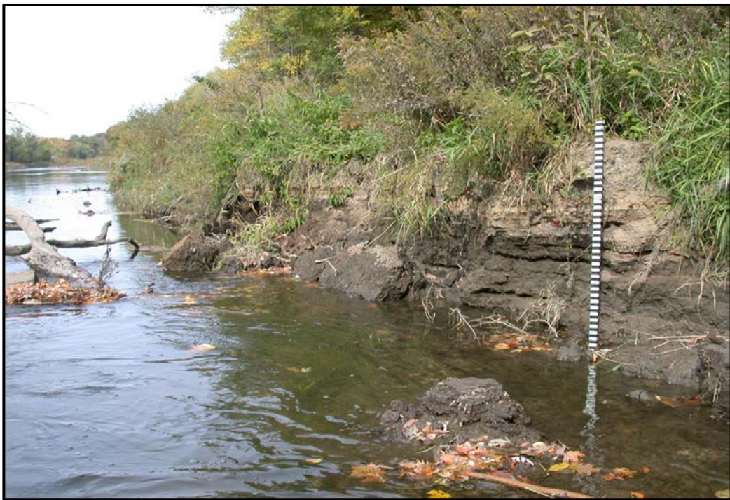
Figure 64. Photographs of large woody debris (LWD) related erosion at transect U-6 (7,056 m ULFD) in October 2012 (Peck personal communication). In both photos flow is from right to left and the scale bar is 1.5 m long. (Top) The extent of the LWD and actively eroding vertical scarp upstream (right) and vegetated bank downstream (left). (Bottom) Close up of the actively eroding bank and recent slump blocks. Note the boils on the stream surface upstream of the LWD.
