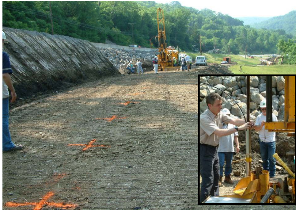
Figure 5.1: JEF-152 Failed Slope under Repair
