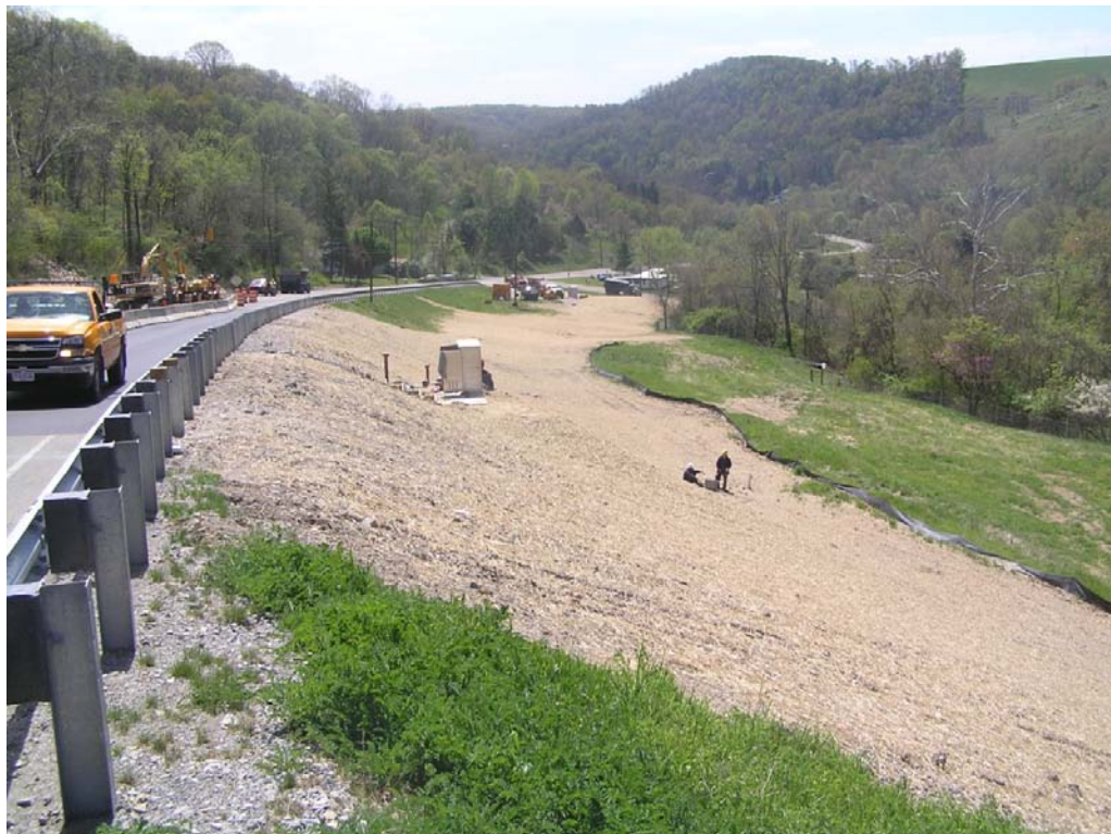
Figure 5.2: The Re-constructed JEF-152 West Embankment
