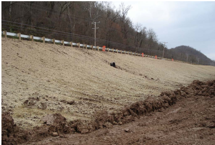
Figure 5.17: The Restored Embankment at WAS-7 Site.
