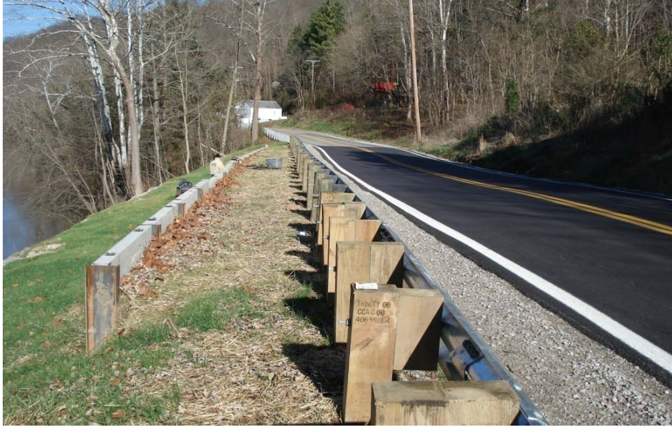
Figure 5.34: A Picture Showing the Restored Slope at MRG-376 Site
