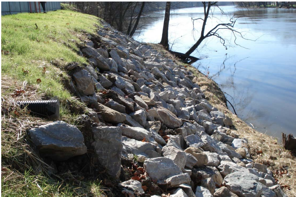
Figure 5.35: A Picture Showing the Rip Rap Placed at the Toe of the Restored Slope at MRG-376 Site
