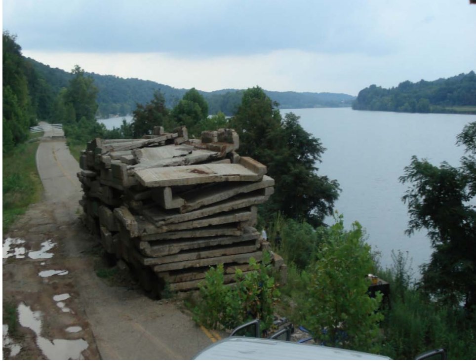
Figure 4.10: A Picture Showing the Surcharge Load Placed at the Test Site
