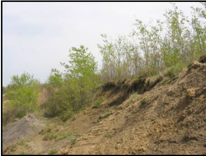
Figure 3.2 Slope with high potential to affect the roadway
