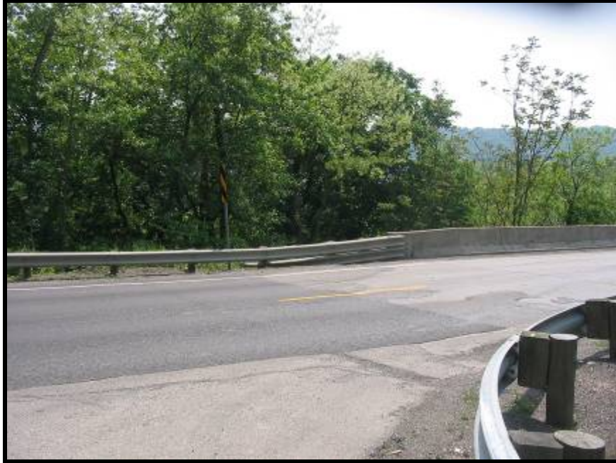
Figure 4.2 Southbound lane direction
