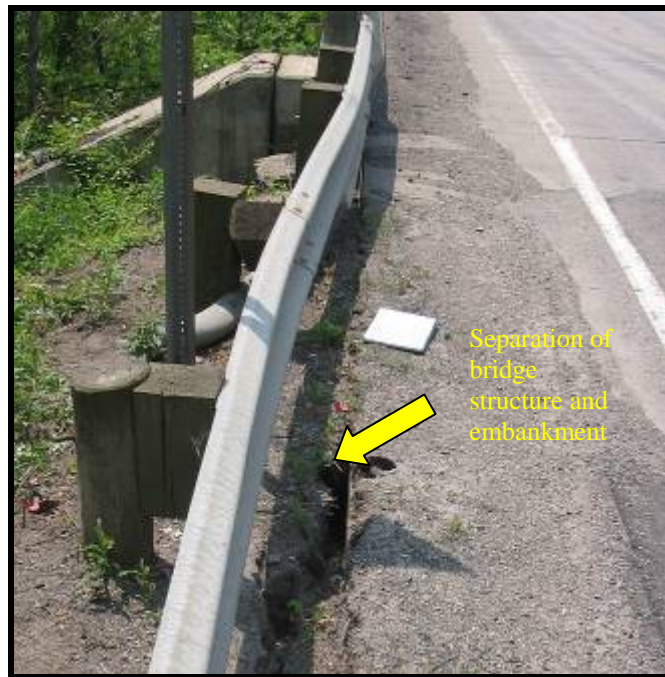
Figure 2.4 Separation of slope and bridge structure
