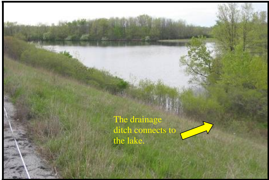
Figure 4.9 Lake at the toe of embankment
