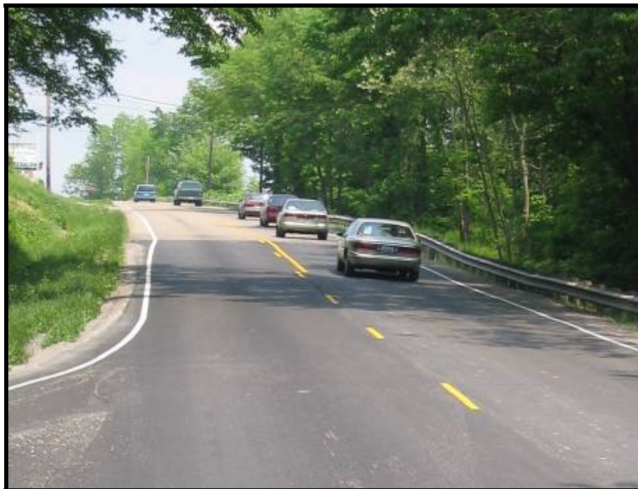
Figure 3.18 A restrict sight distance due to vertical curve
