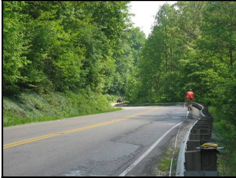
Figure 3.17 Example of a horizontal curve that could hide the slope hazard on the road ahead
