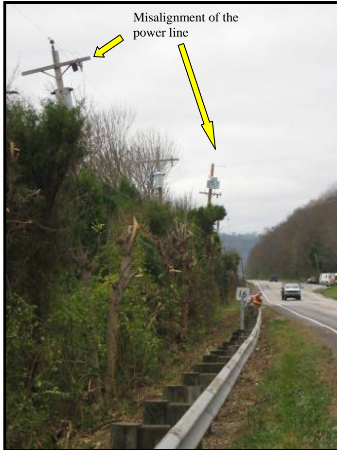
Figure 2.2 Misalignment of power line
